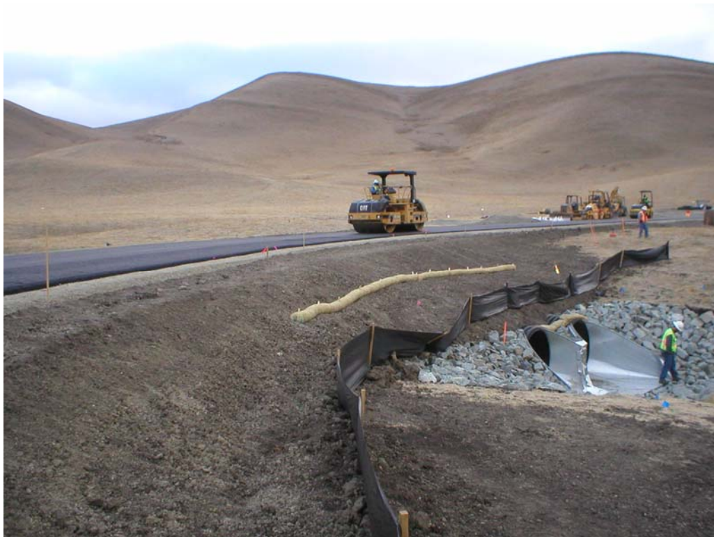
Figure 4 – Paving activities on Road 6, November 11 th .
