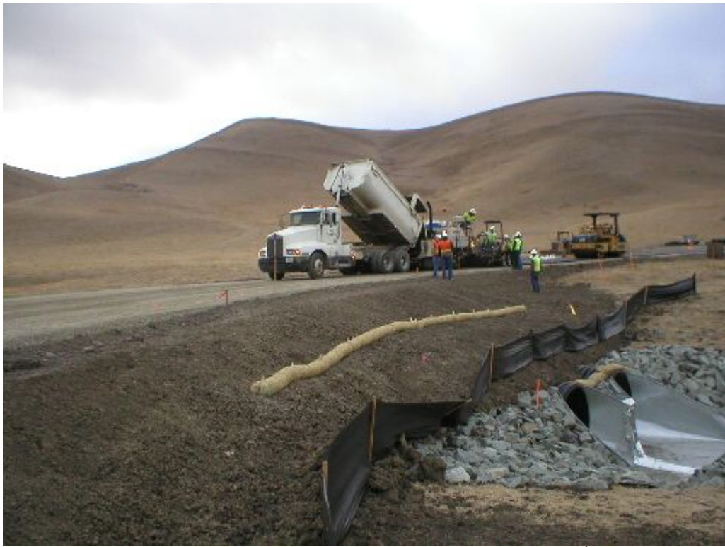
Figure 3 – Paving activities on Road 6, November 11 th .
