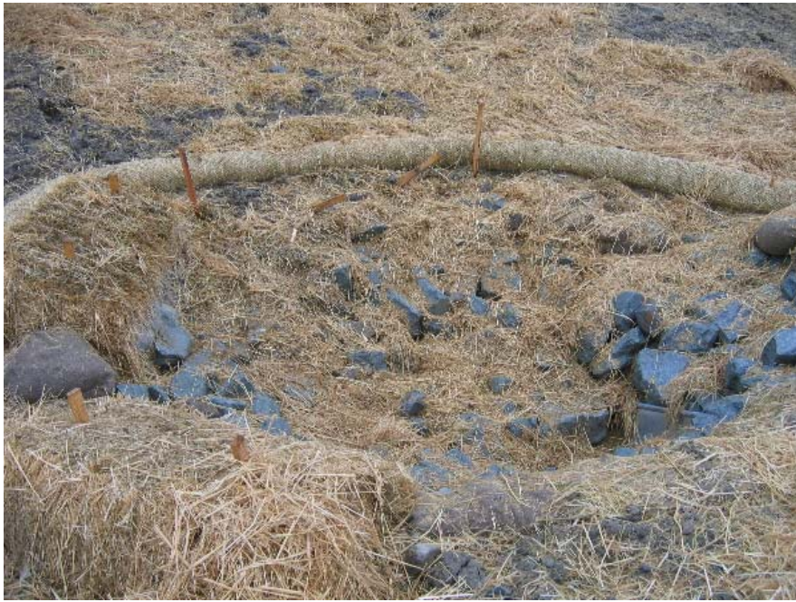
Figure 4 – Previously clogged culvert after repairs along the MSA Road, November 30, 2005.
