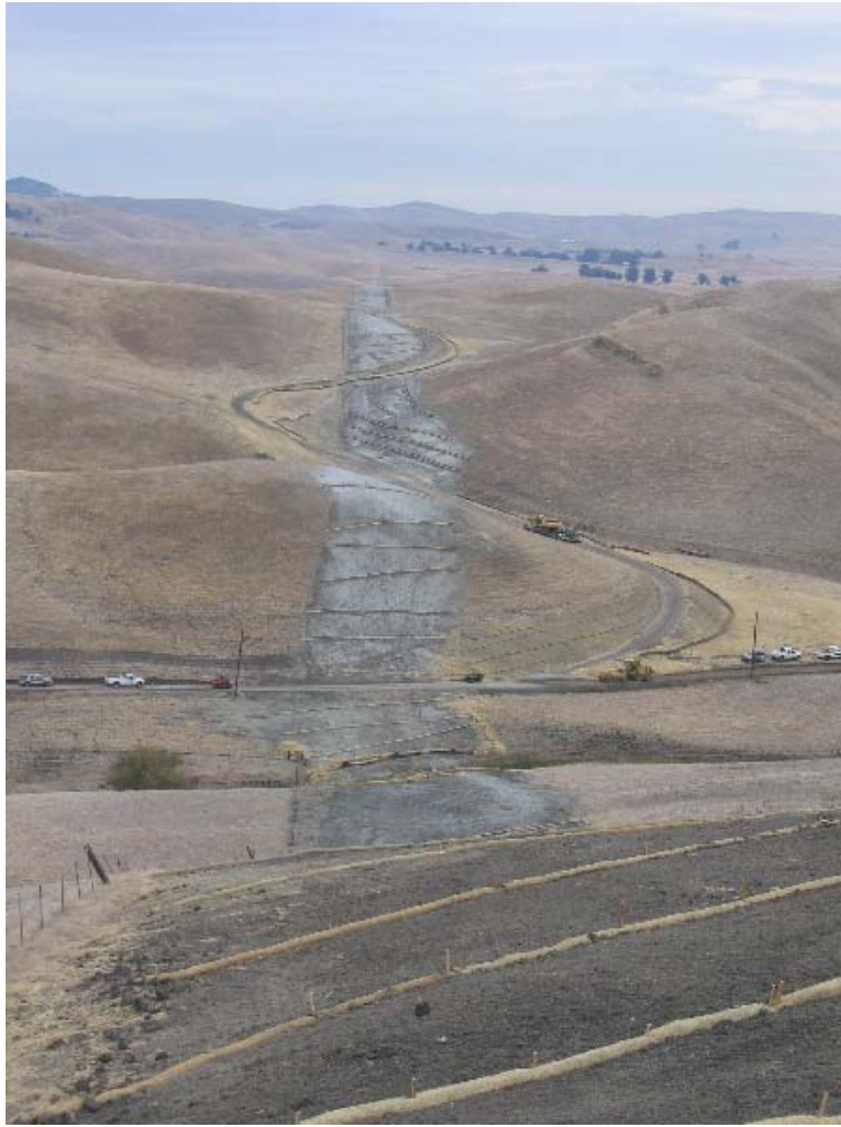
Figure 1 – Trench line extending from the Transition Station and Road 7, November 30.
