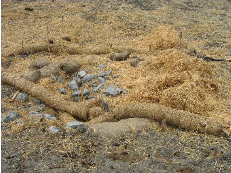
Figure 3 – Clogged culvert in need of repair along the MSA Road, November 28, 2005.
