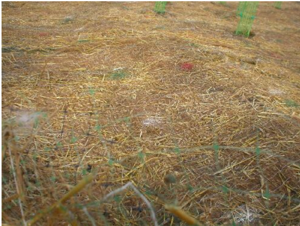
Figure 4 – Close up view of the monofilament matting the Mitigation Area, December 14, 2005. Note the green grid top layer. Hay is sandwiched in between two such layers.
