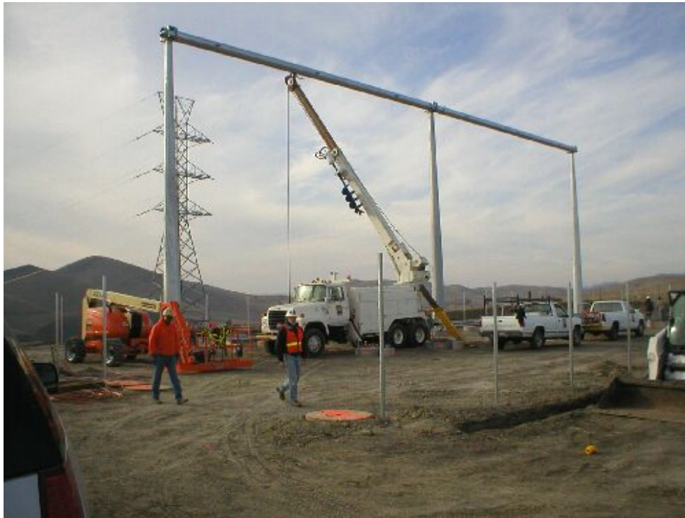
Figure 1 – Crews have installed the frame structure at the Transition Station, December 15, 2005.
