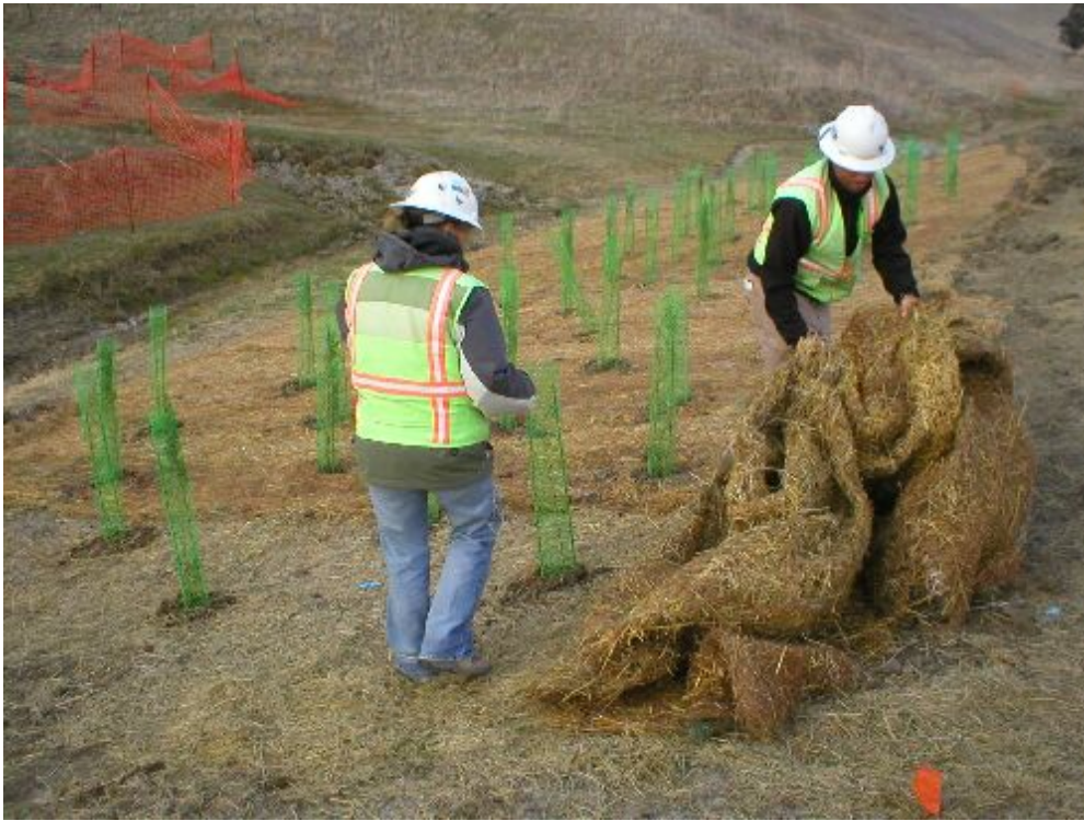
Figure 5 – PG&E EI/Opus removing the monofilament matting installation, December 14, 2005.
