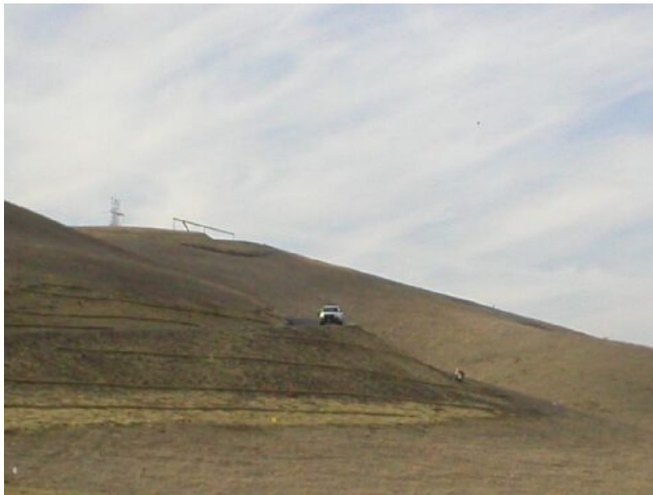
Figure 2 – Granite was on-site conducting erosion control maintenance along Road 6 at a culvert, December 15, 2005.
