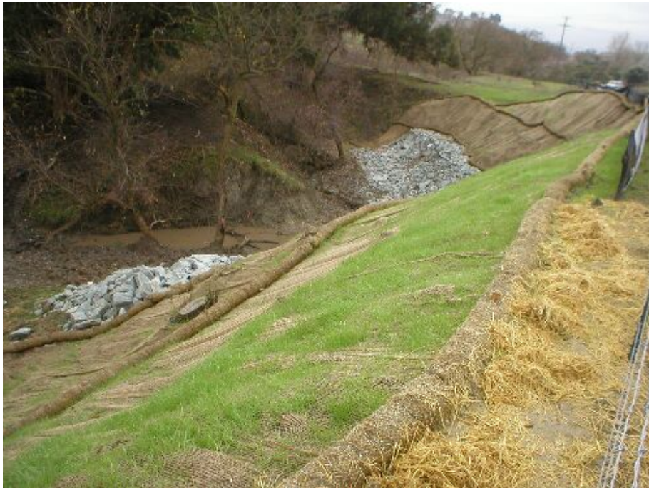
Figure 4 – Good grass growth above the bank stabilization area along Moller Road, December 29, 2005.
