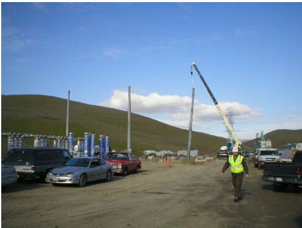
Figure 6 – Tower assembly at the North Dublin Substation, January 25, 2006.
