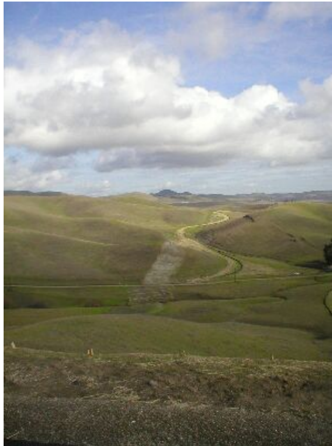
Figure 4 – Road 7 - Note the areas of construction without grass cover, January 27, 2006.
