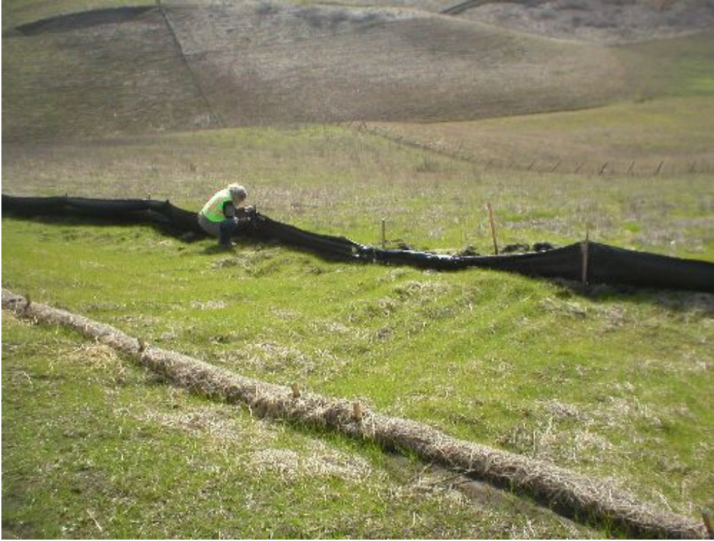
Figure 1 – Sediment fence repair down slope from the Transition Station, January 27, 2006.
