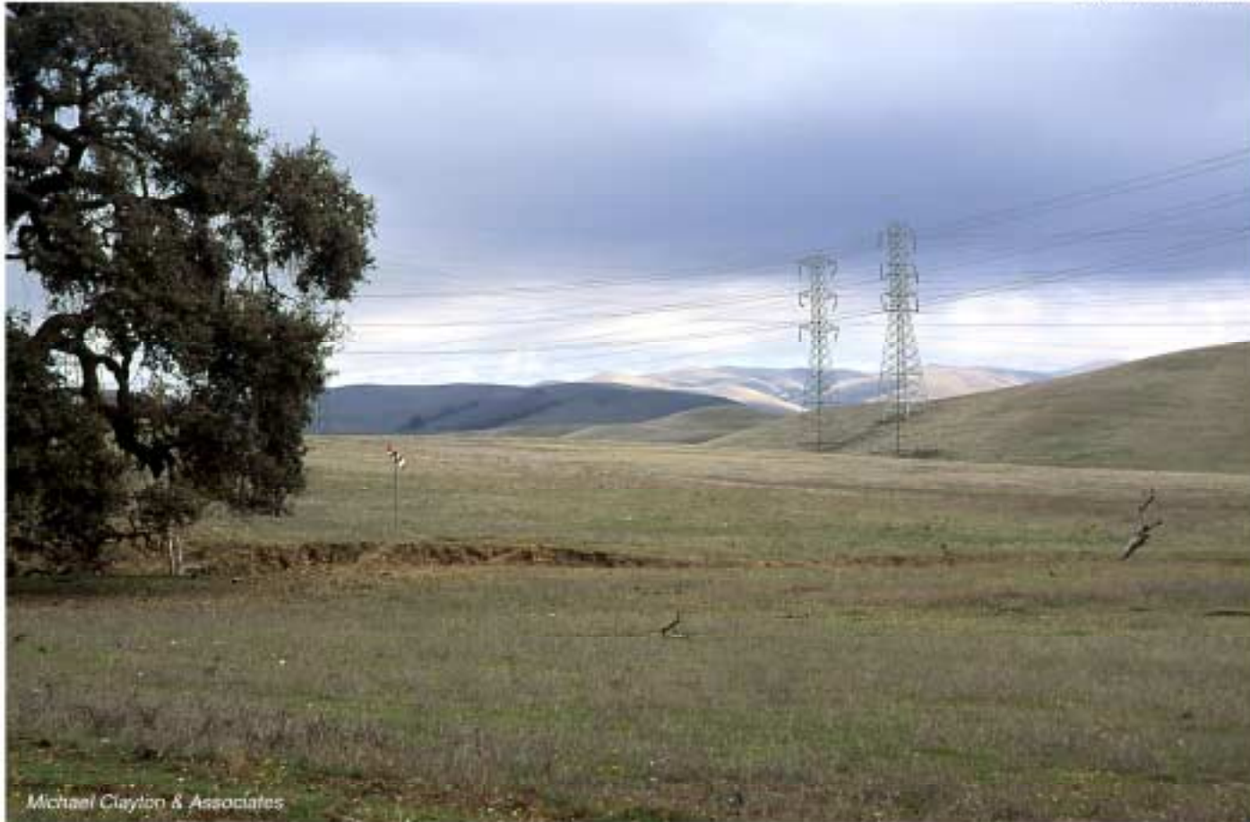
The existing view to the southeast toward Switching Station Site No. 1 in the Tesla-Newark Corridor. The proposed site would be located in the center of the photograph between the Stanislaus Line on the north (behind the tree) and the Contra Costa-Newark Line to the south (shown in the right of the photograph). Switching Station Site No. 1 Tesla-Newark Corridor Tri-Valley 2002 Capacity Increase Project EIR FIGURE C.13-1
