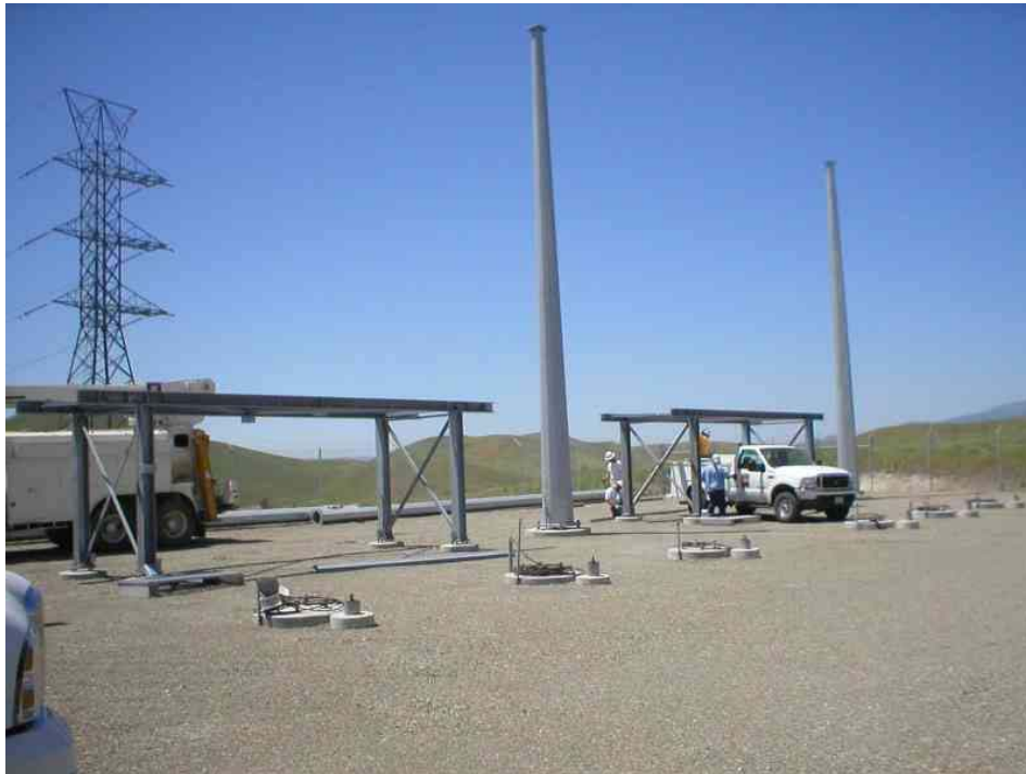
Figure 2 – Wilson crew re-erecting the Transition Station structure, May 15, 2006.
