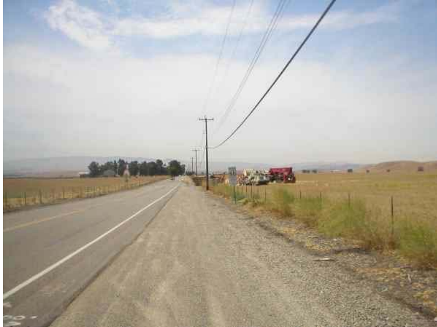
Figure 1 – Overturned cable reel and crane remain at the Vault 3 accident location. June 26, 2006.
