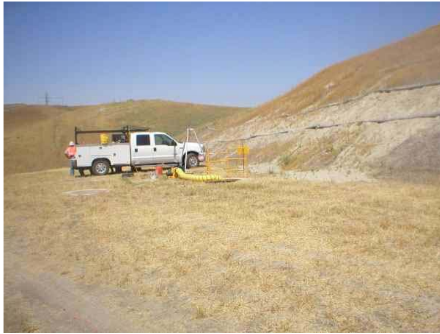
Figure 3 – Jensen PreCast crews conducting racking at Vault 7. June 26, 2006.
