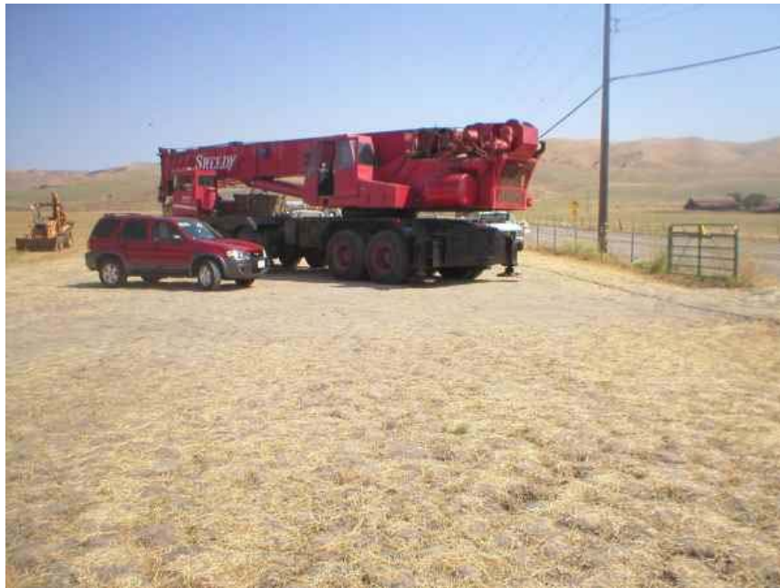
Figure 2 – New crane brought to the Vault 3 location. June 26, 2006.
