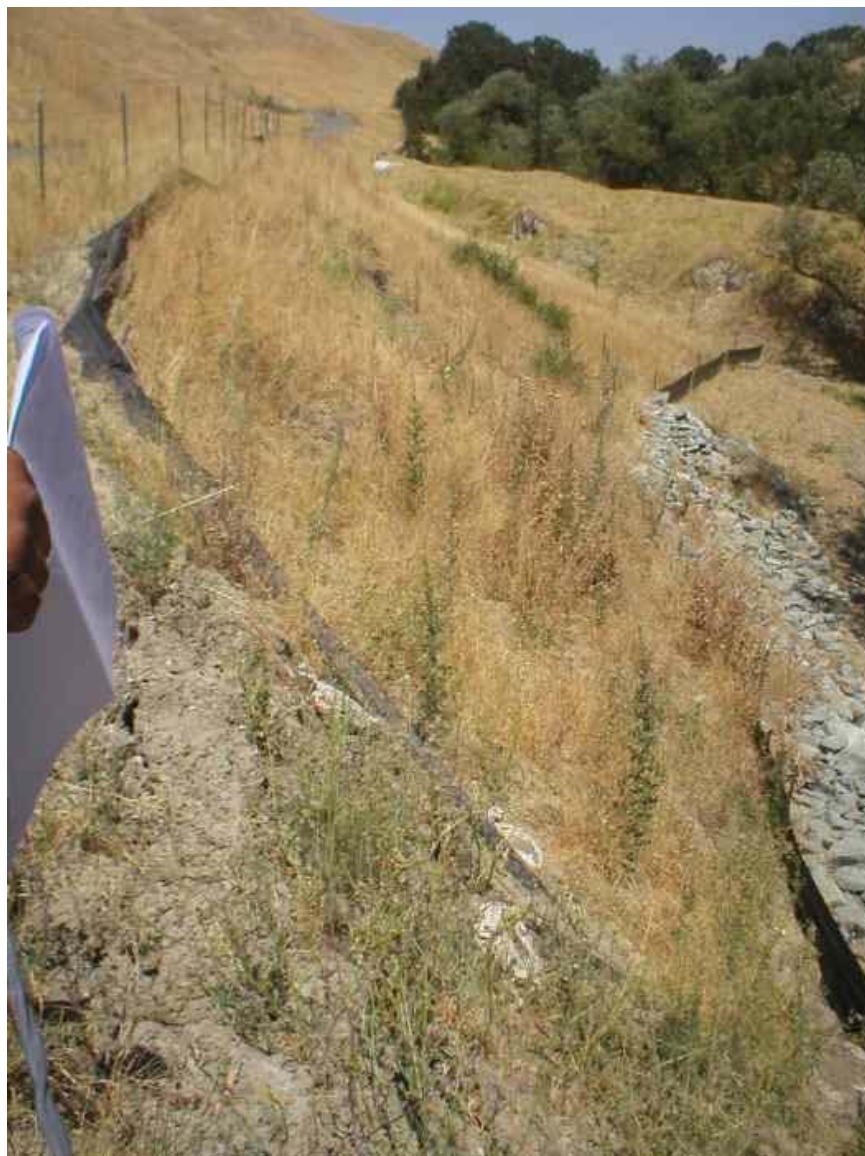
Figure 1 – Tassajara Creek bank stabilization area slated for restoration. August 3, 2006.
