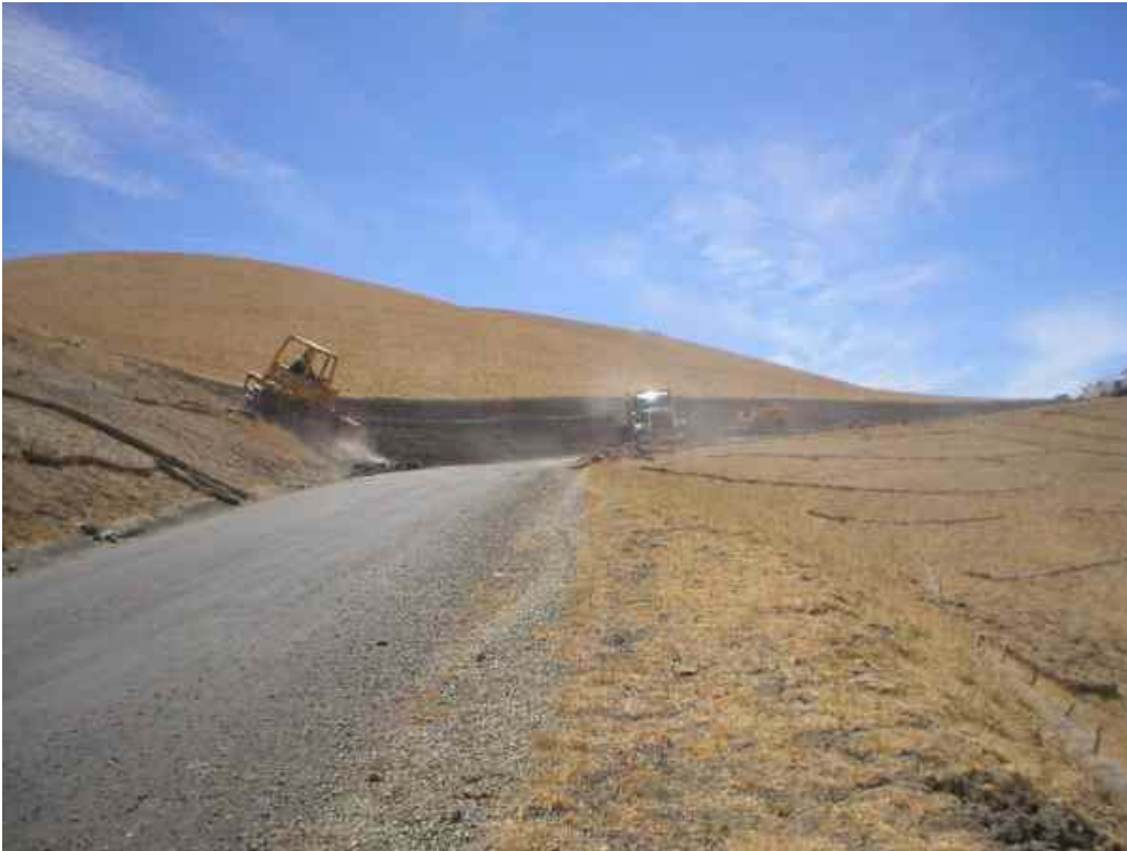
Figure 2 – Restoration work on the previously slumped section upslope of Road 6, August 23, 2006.
