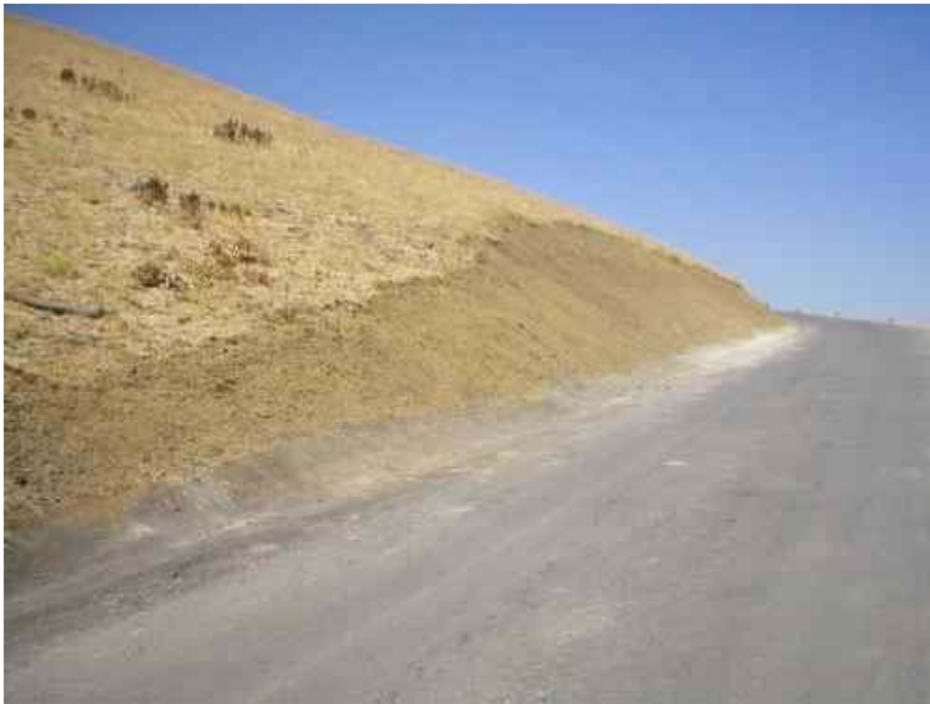
Figure 5 – NVC crews re-contoured and seeded a side slope along Road 6, September 7, 2006.
