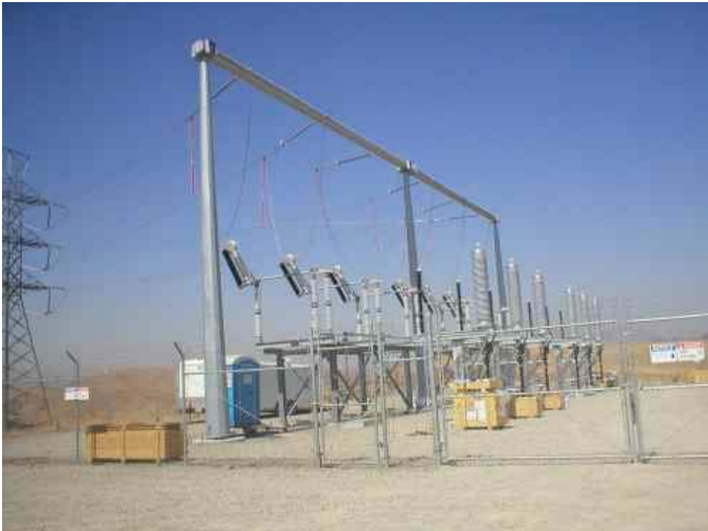
Figure 2 – Transition Station, September 7, 2006.
