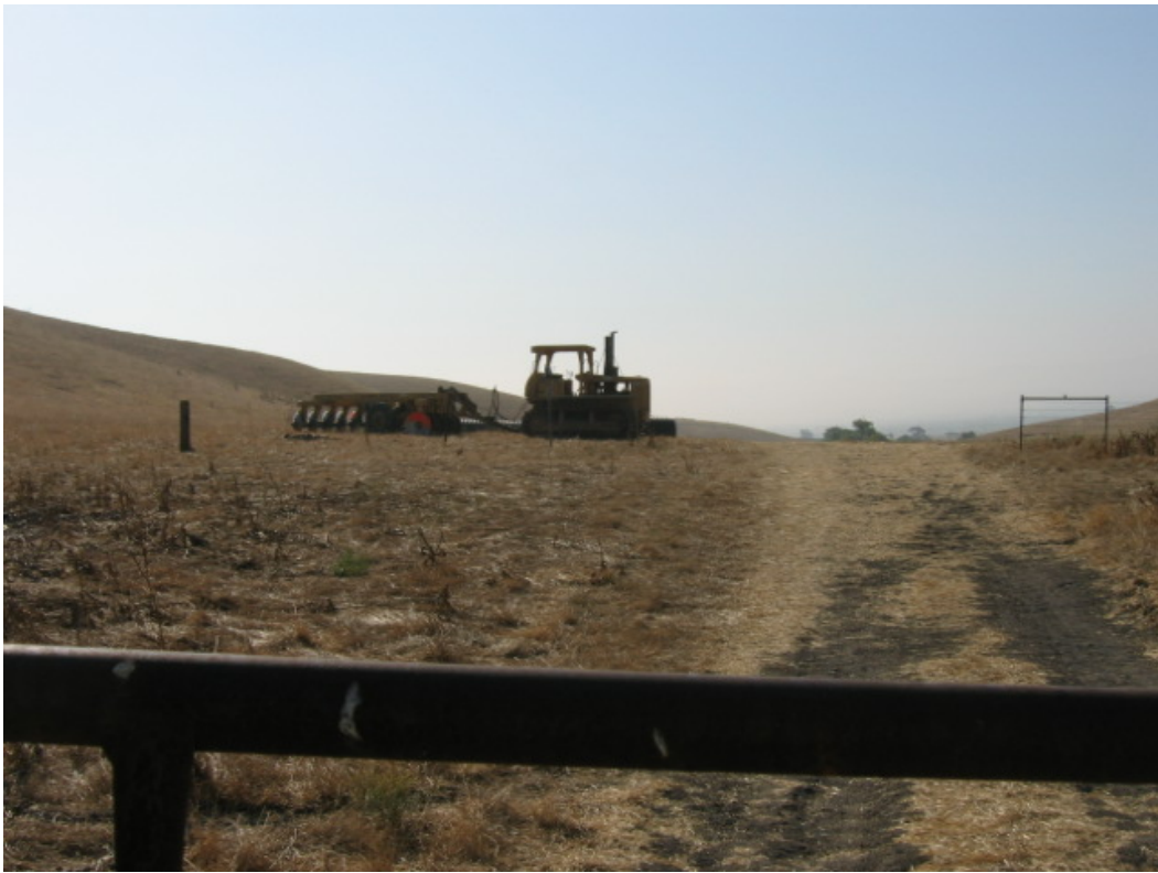
Figure 5 – Equipment staged outside ROW near Access Road 5. Phase Three, July 28, 2005.
