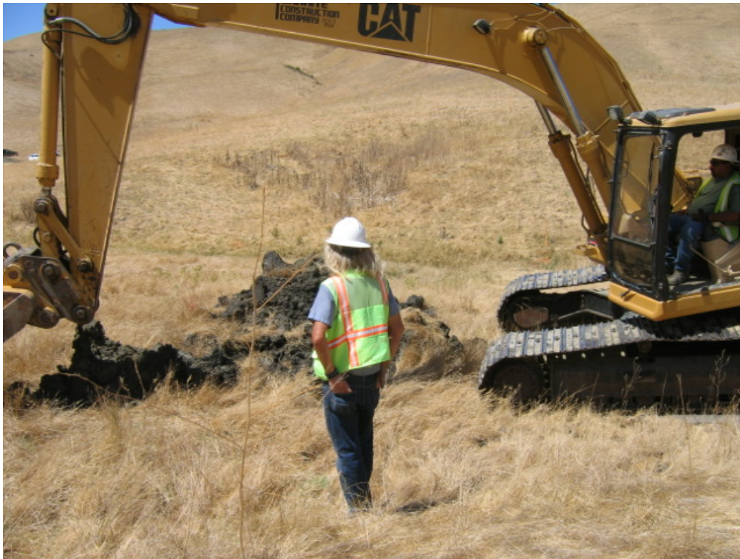
Figure 3 – A PG&E EU monitors excavation within the mitigation pond area, August 24, 2005.
