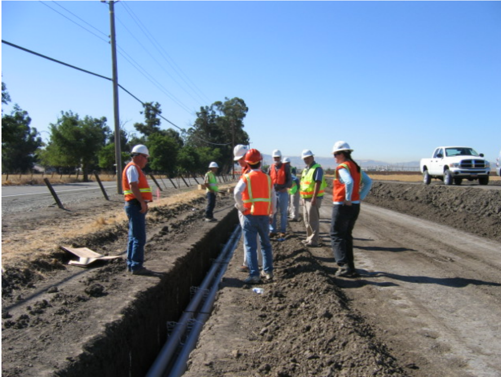
Figure 1 – CPUC staff inspecting trenching along North Livermore Ave., August 23, 2005.
