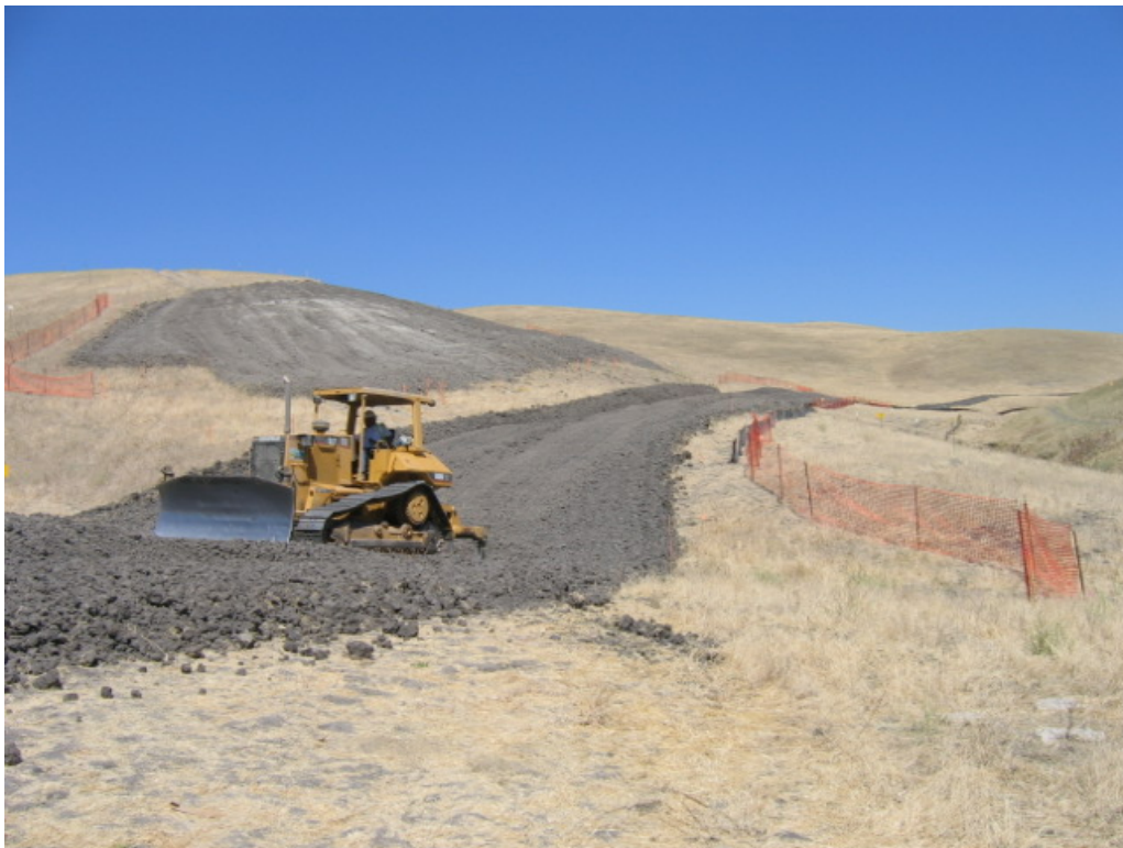
Figure 2 – Construction of Access Road 7, August 24, 2005.
