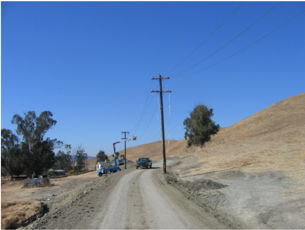
Figure 3 – Stringing taking place along Moller Road, September 28, 2005.
