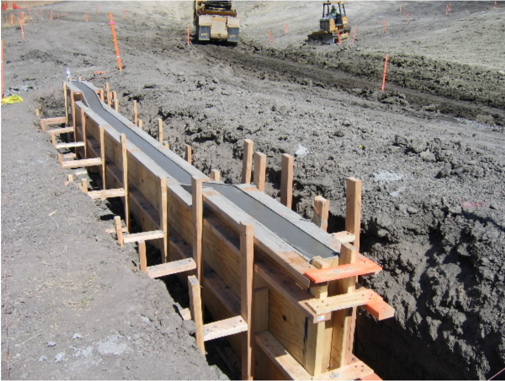
Figure 1 – Spillway construction at the Mitigation Pond site, September 27, 2005.
