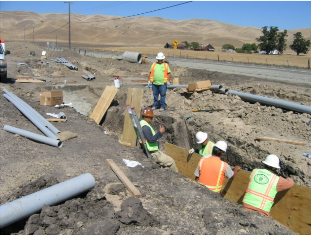
Figure 2 – Crews conducting tie-ins along North Livermore Avenue, September 28, 2005.
