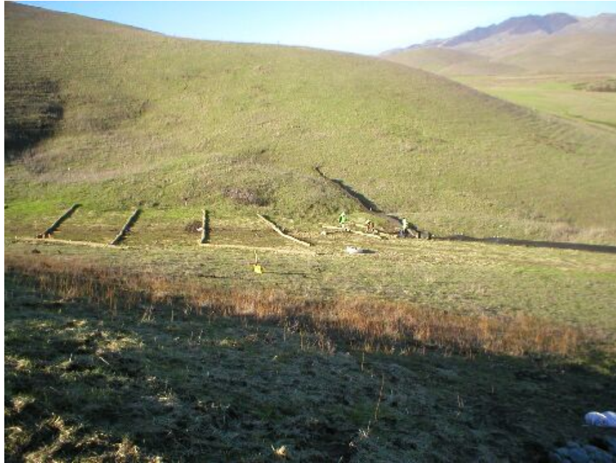
Figure 1 – Erosion down slope of Road 6, January 4, 2006.
