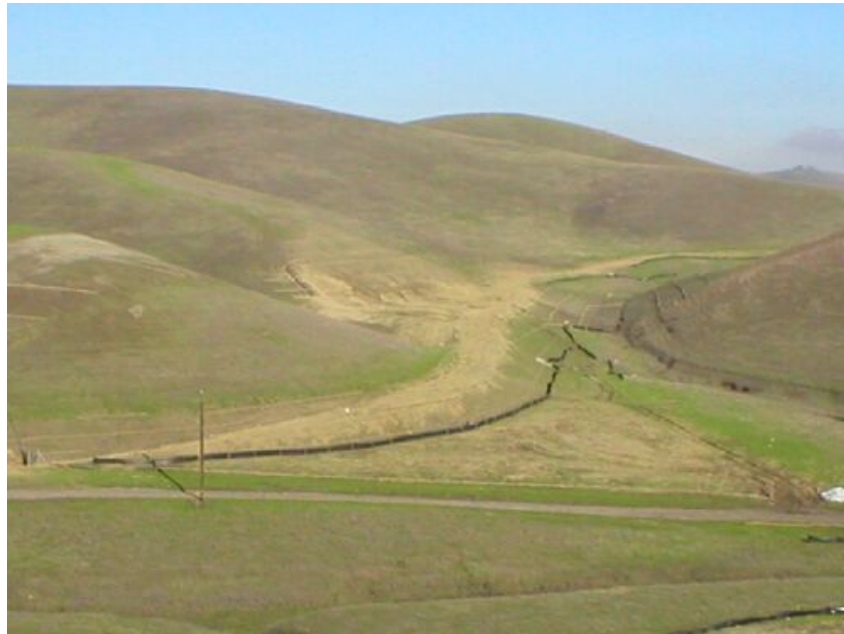
Figure 2 – Road 7 landslide area, January 4, 2006.
