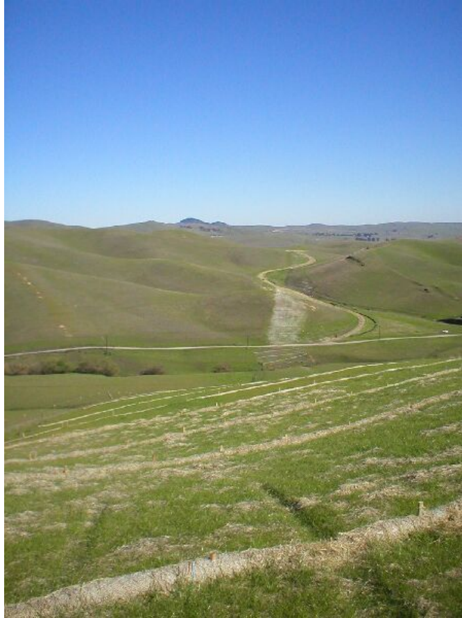
Figure 1 – View of the underground alignment and Road 7 extending from the Transition Station – February 21, 2006.
