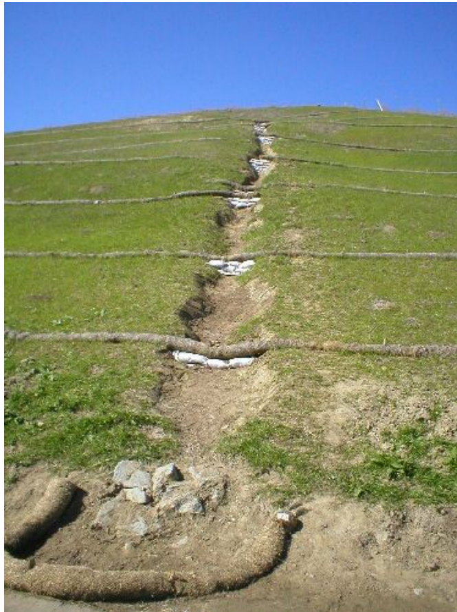
Figure 2 – Re-contoured and compacted v-ditch along Moller Road, February 21, 2006.
