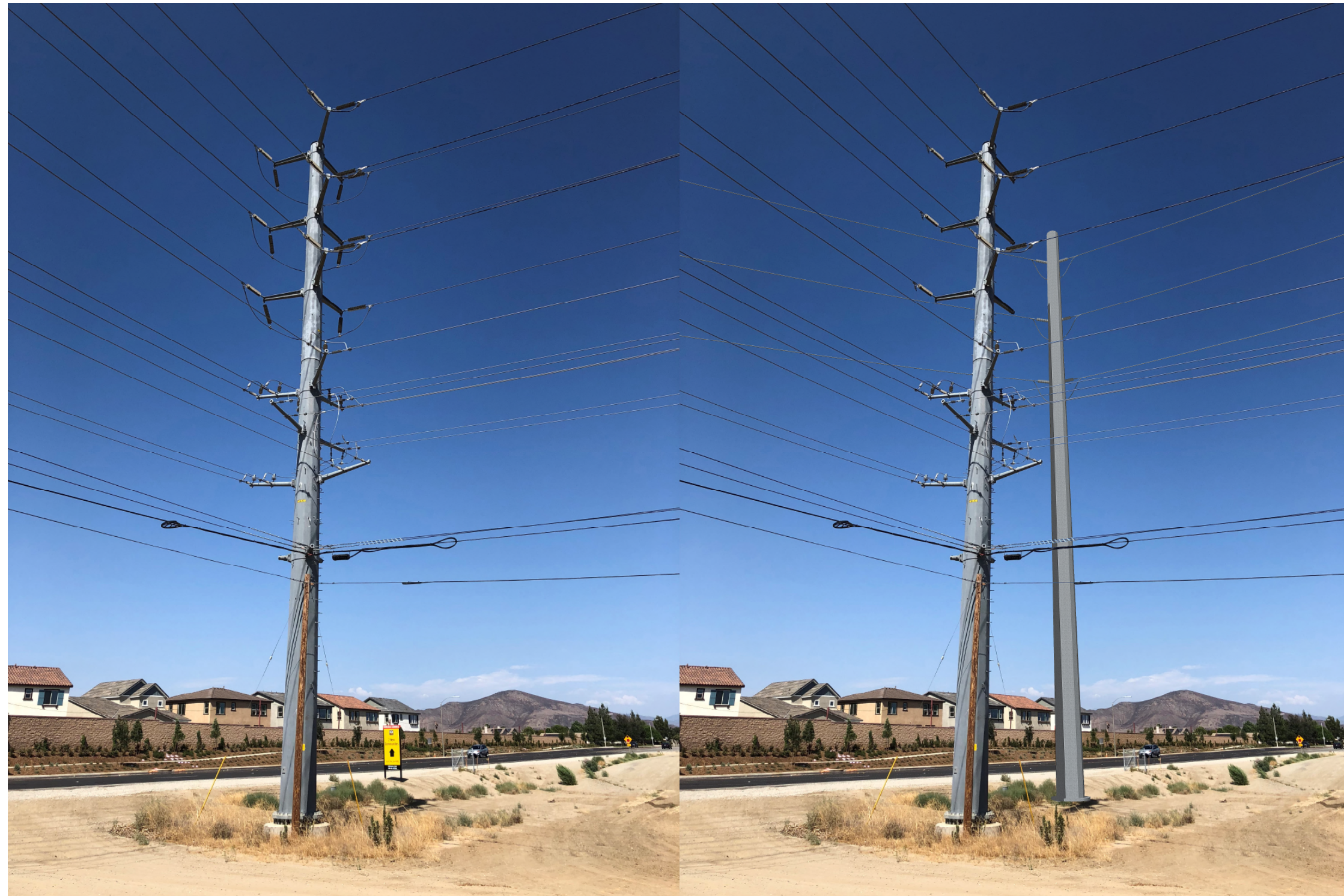
Simulated view depicting a light gray dulled galvanized TSP at intersection of Leon Rd. and Benton Rd. (Left: Existing conditions, Right: Simulation of new proposed TSP)
