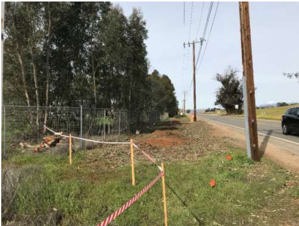
Photo 2 – Vegetation removal was completed at Vegetation Management Area #6.
