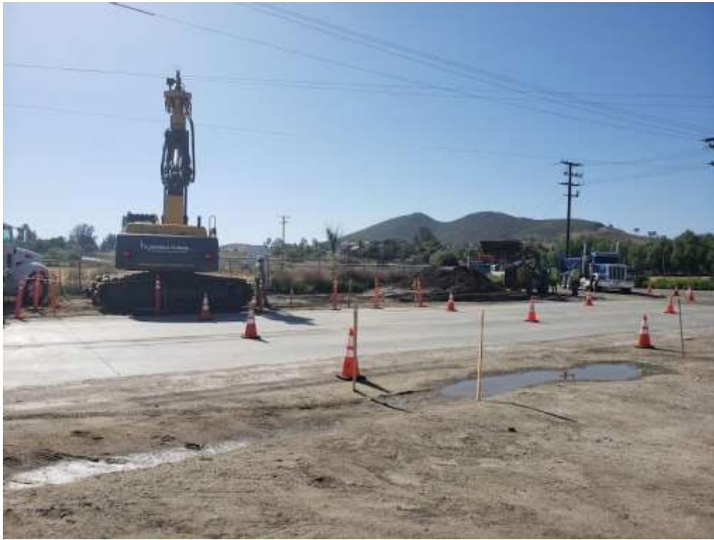
Photo 1 – Foundation drilling at Construction Area UNK 154 (May 29, 2019)
