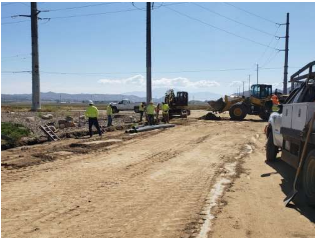
Photo 2 – Underground trenching from Valley Substation to Meniffee Road (May 29, 2019).
