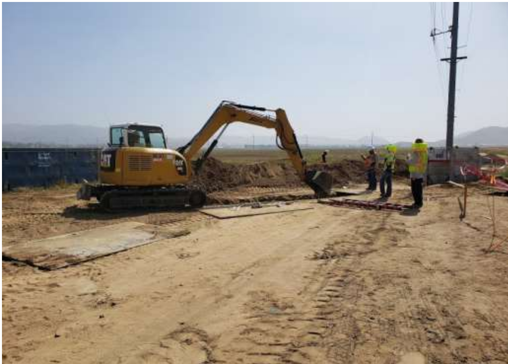
Photo 2 – Underground trenching from Menifee Road to Construction Area UNK250 (June 18, 2019).
