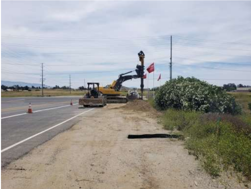
Photo 1 – Foundation drilling at Construction Area UNK247 (June 11, 2019).
