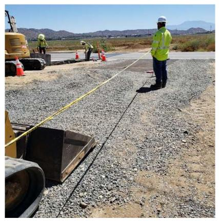
Photo 4 – SWPPP TC-1 required stabilized construction entrance on west side of Menifee Road near Valley Substation (July 2, 2019).
