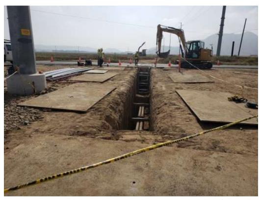
Photo 2 – Underground trenching and conduit installation under Menifee Road (June 26, 2019).
