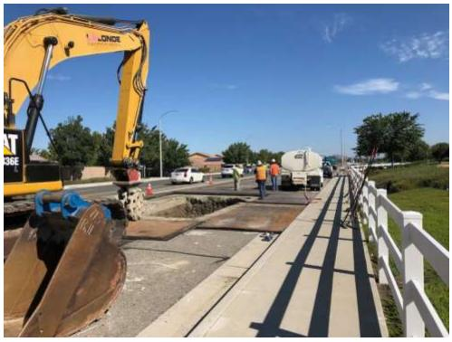
Photo 1 – Vault excavation on the southern underground (September 6, 2019).
