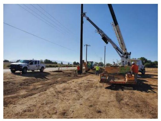
Photo 2 – Setting wood pole at Construction Area UNK183 (October 2, 2019).
