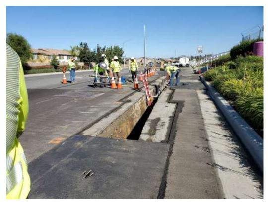
Photo 1 – Conduit installation on the southern underground (October 9, 2019).
