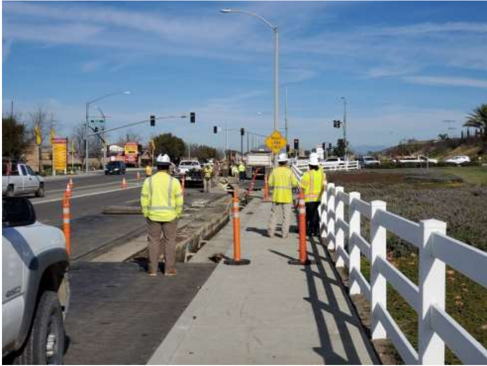
Photo 1 – Trenching and conduit installation on the southern underground (January 15, 2020).
