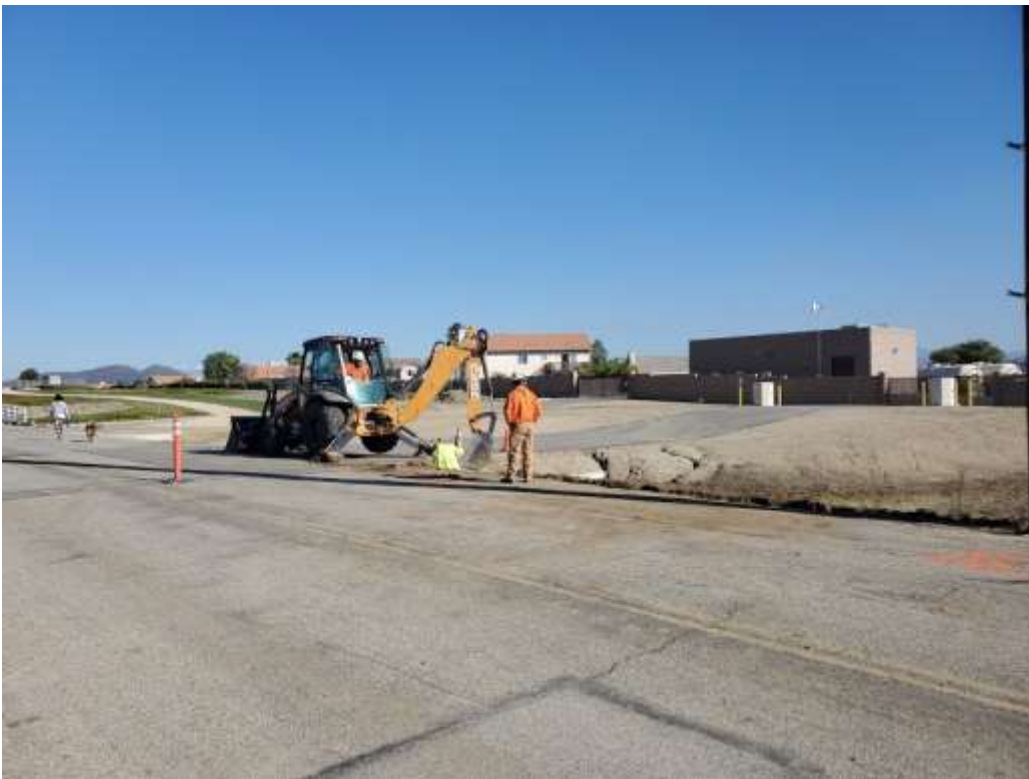
Photo 4 – Trenching for conduit installation at Construction Area UNK224 (January 15, 2020).
