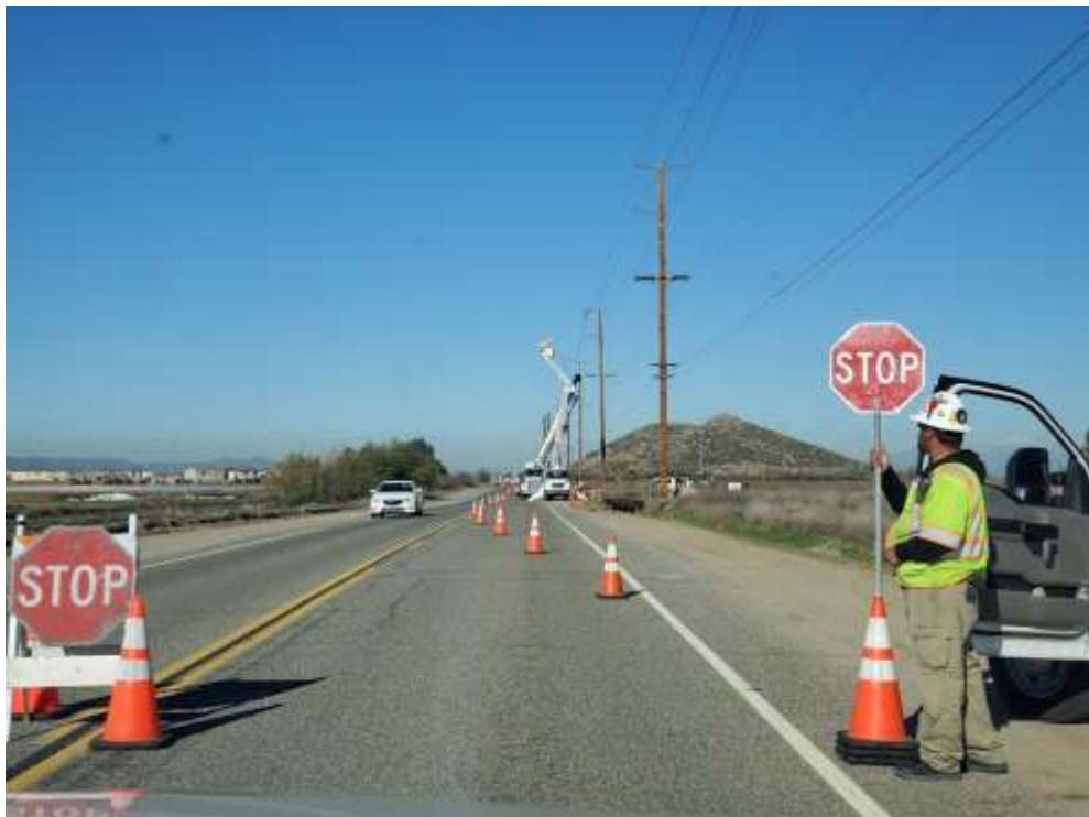
Photo 2 – Wire stringing activities at Construction Areas UNK03 to UNK09 with traffic control in place (January 8, 2020).
