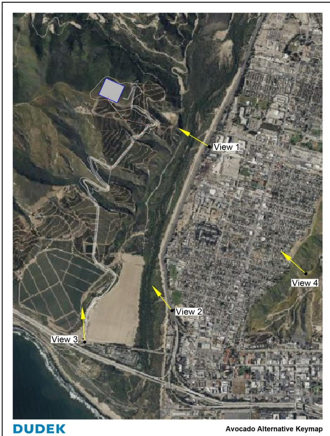
Exhibit 1-10: Avocado Site overview showing Views 1–4
