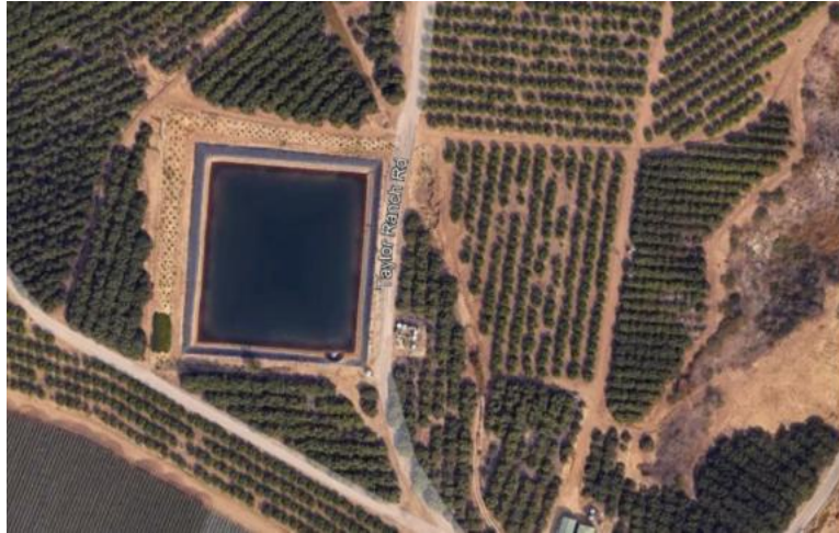
Exhibit 1-9: Avocado orchard support infrastructure, including irrigation equipment and retention pond, along Taylor Ranch Road (via Google Earth, May 2025)
