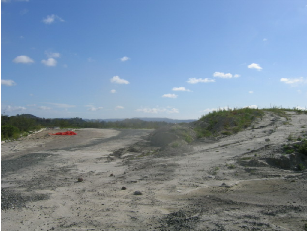
Photo 1: Spoil pile in laydown area behind the Viejo Substation that needs to be removed (mound in center of frame).
