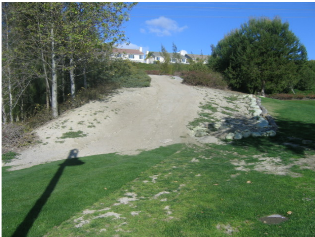
Photo 4: Restoration of a pre-existing access road near Olympiad Park.
