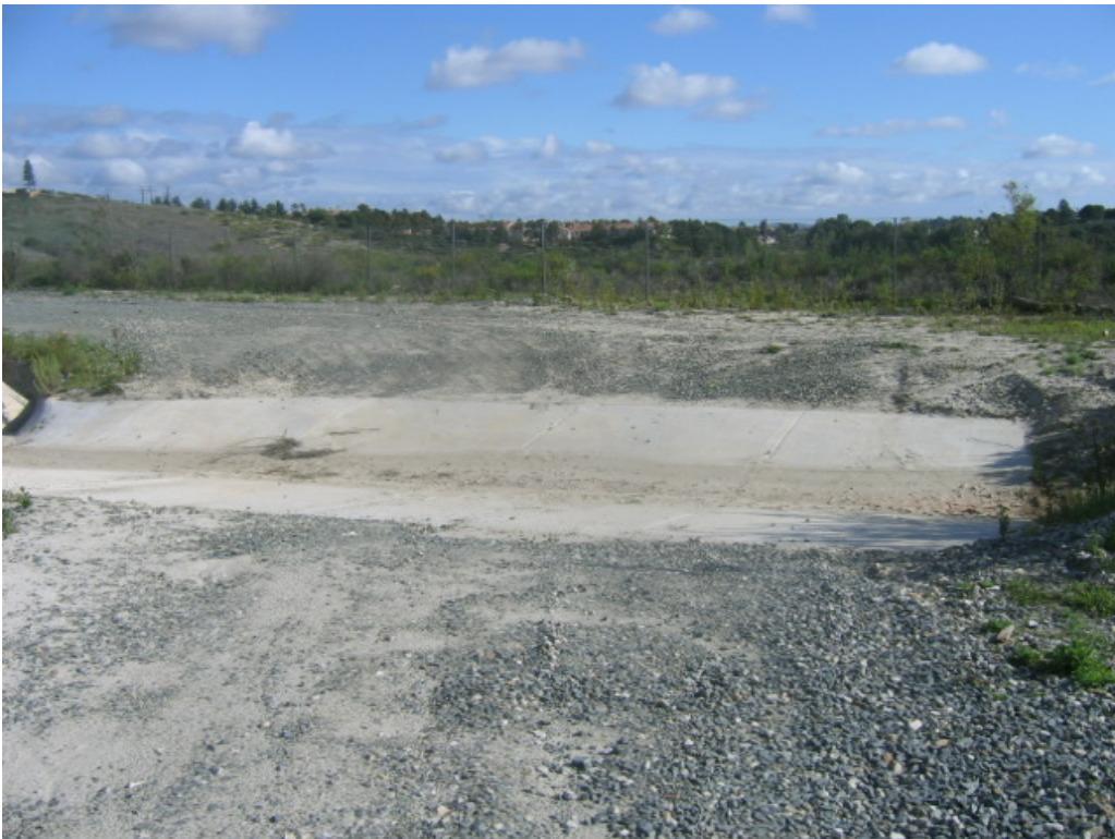
Photo 2: Wet-crossing on access road behind Viejo Substation.
