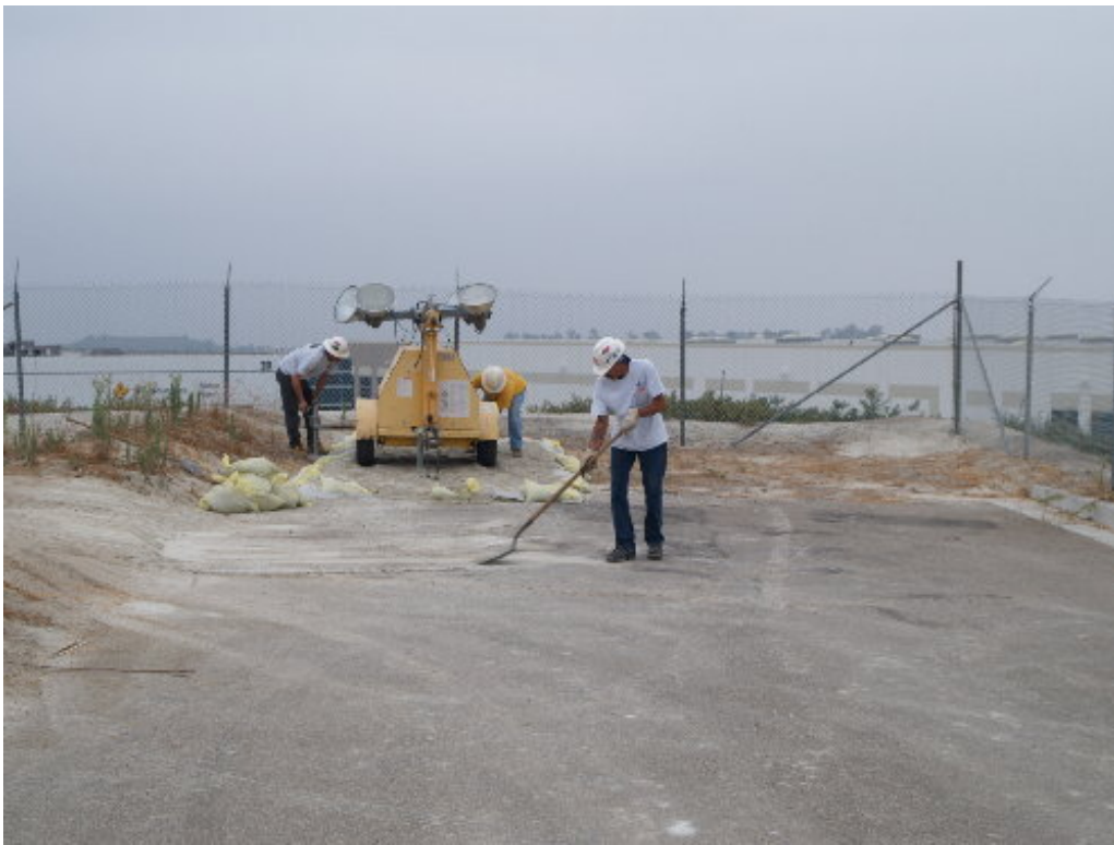
Figure 2 – Containment berm for the portable light plant filled with sand (contractor will place additional layer of sandbags to increase capacity of berm).
