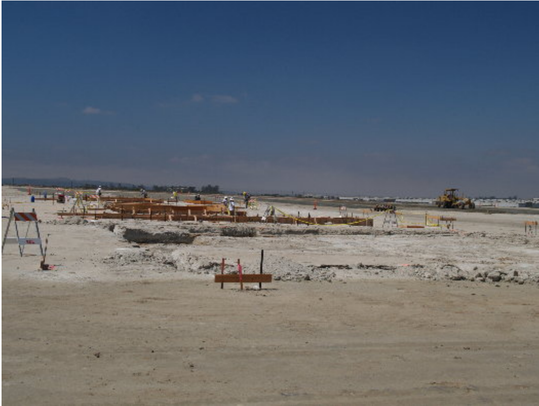
Figure 3 – Crews starting construction of form work for building foundations.
