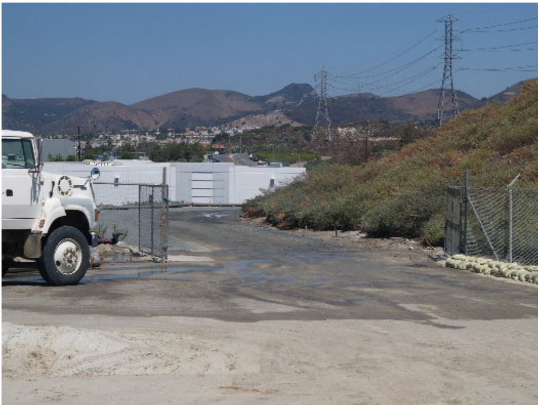
Figure 4 – SCE plans to submit a variance request for cutting the toe of the slope on the access road to allow for larger tractor trailers.
