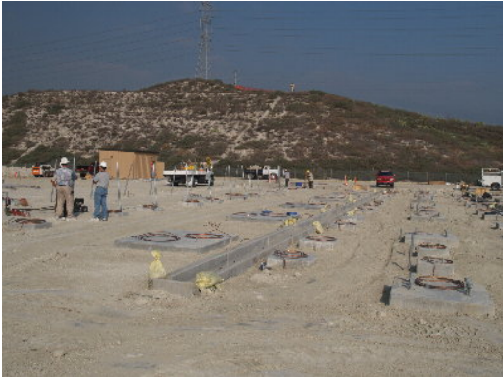
Figure 3 – A crew worked on attaching foundations to the grounding grid.
