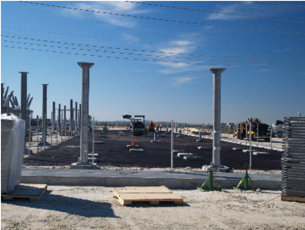
Figure 3 – A crew worked to lay asphalt north of MEER #1.
