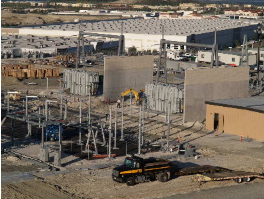
Figure 1 – Crews prepared A transformers once they were set onto the pads.
