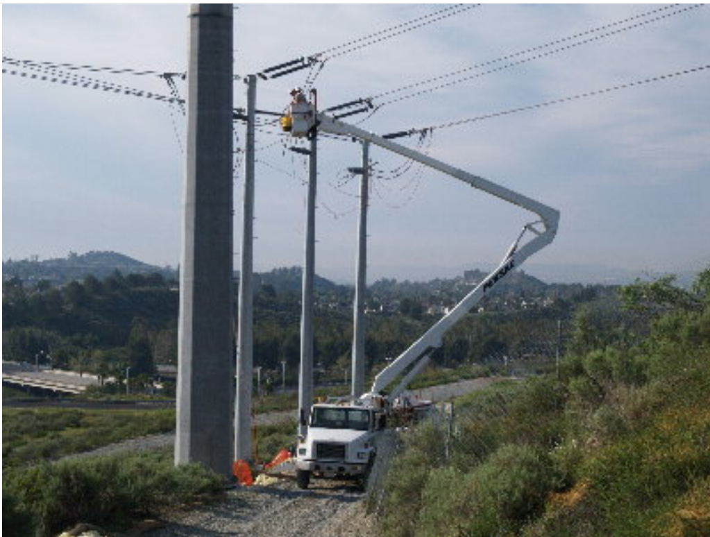
Figure 4 – The transmission line crews worked in man-lifts to attach cable to the insulators.
