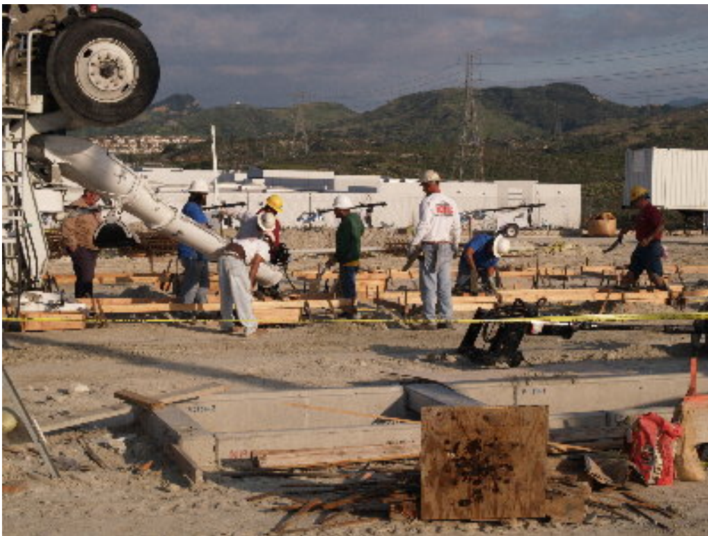
Figure 2 – The 12 kV foundations were poured and the anchor bolts set.
