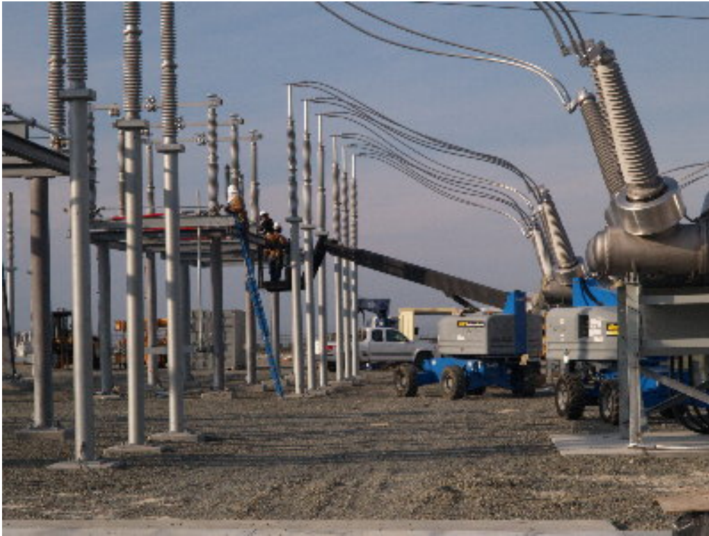
Figure 1 – A small crew worked with lifts to prepare the 220 kV circuits.
