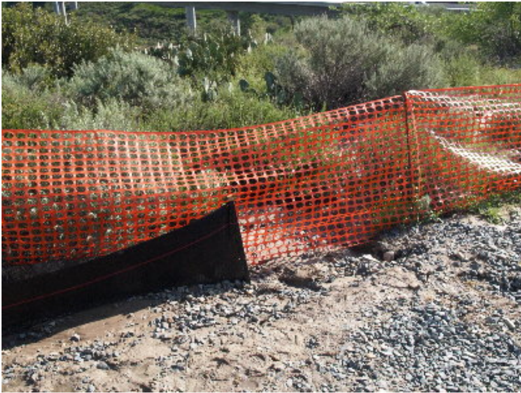
Figure 5 – The silt fencing on the southeastern access road on the 220 kV segment outlets directly to the protected habitat.
