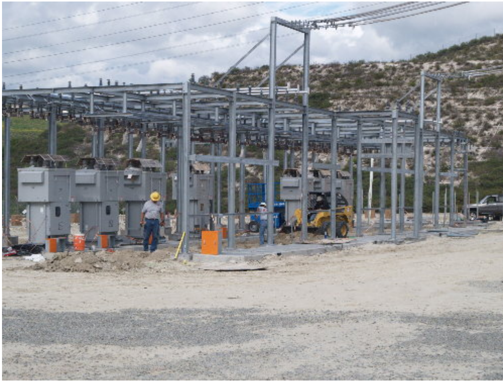
Figure 5 – NRG worked to connect the 12 kV structures to the grounding grid.
