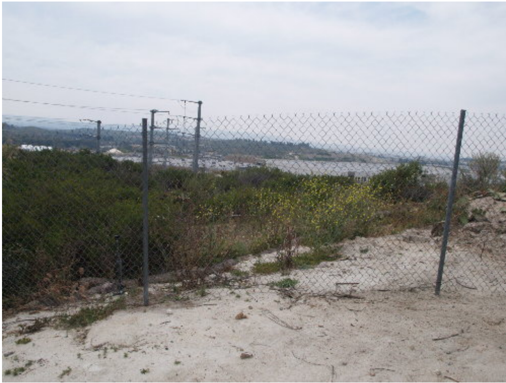
Figure 5 – The CPUC EM reminded SCE to remove invasive non-native plants from the 220 kV right-of-way, adjacent to the native habitat.
