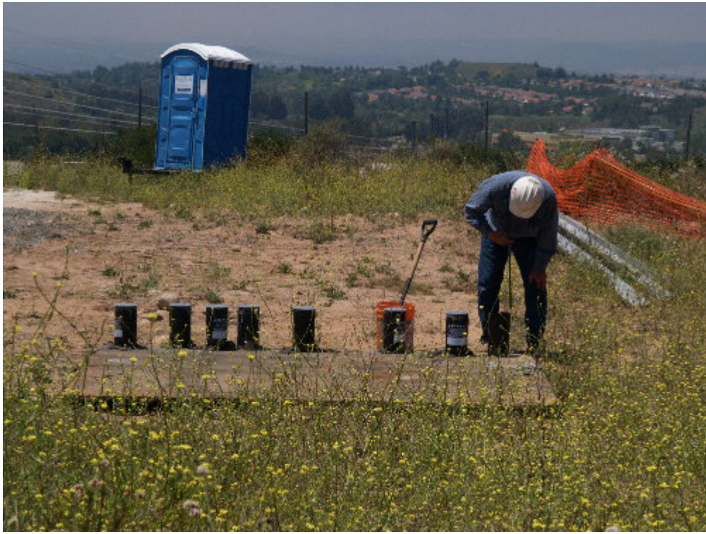
Figure 5 – Each batch of concrete is inspected and samples collected for testing.
