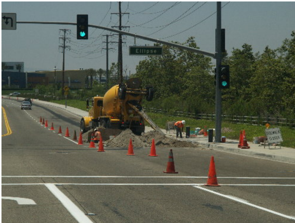
Figure 3 – Arizona Pipeline installed the vents and vent piping for the 12 kV vaults.
