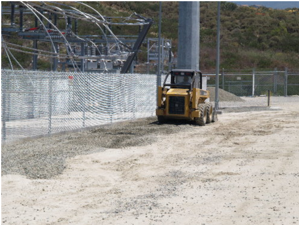
Figure 2 – Rock was placed around completed structures within the substation site.
