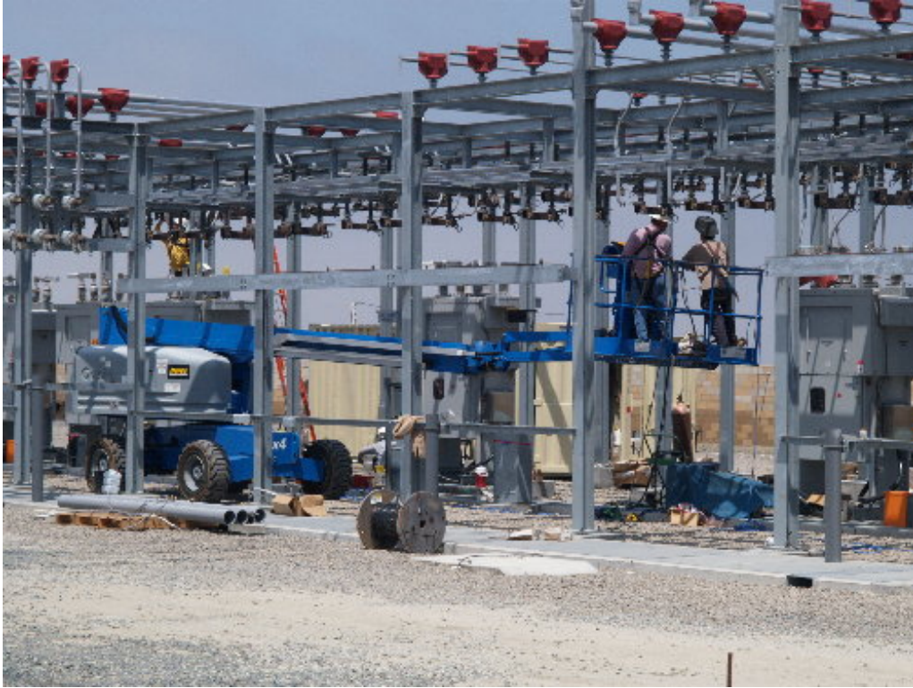
Figure 1 – NRG continued working on the 12 kV portion of the substation.
