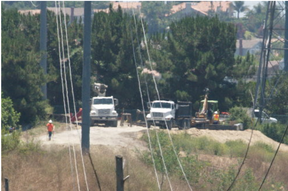
Figure 3 – Crews worked at H-Structure 8 to prepare for concrete pouring.
