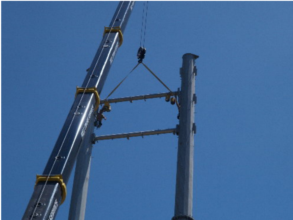
Figure 4 – Workers align and attach the cross members on H-Structure 9.
