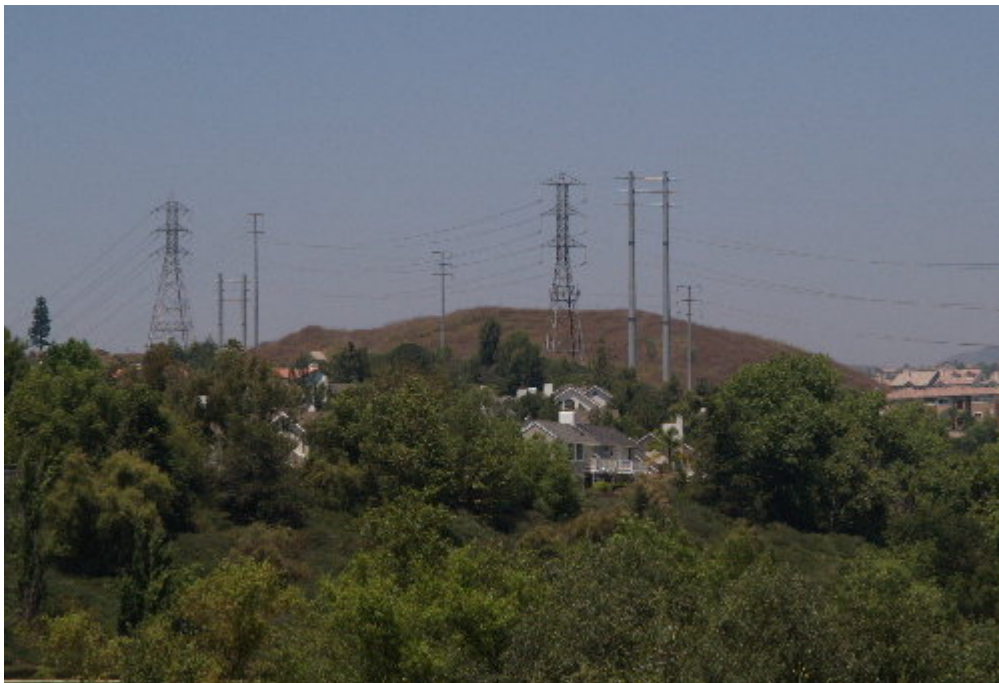
Figure 4 – Raised H-Structures 9 and 10, looking to the north. H-Structure 9 is in the foreground.
