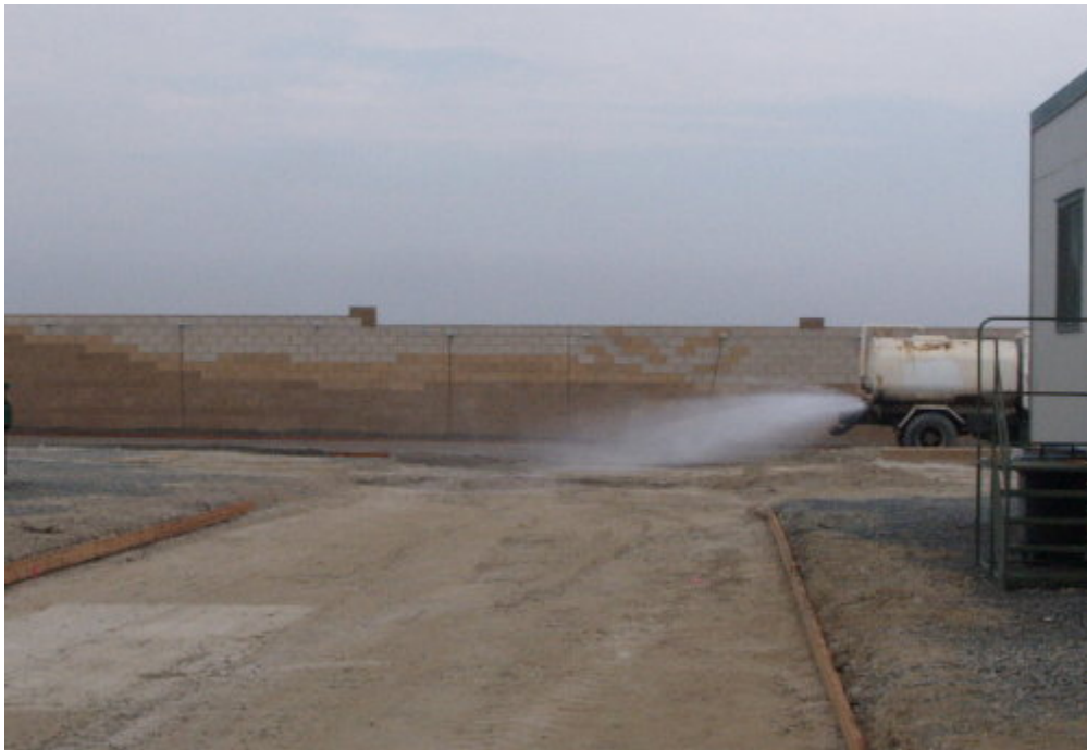
Figure 2 – A water truck was used to control dust during the site visit.
