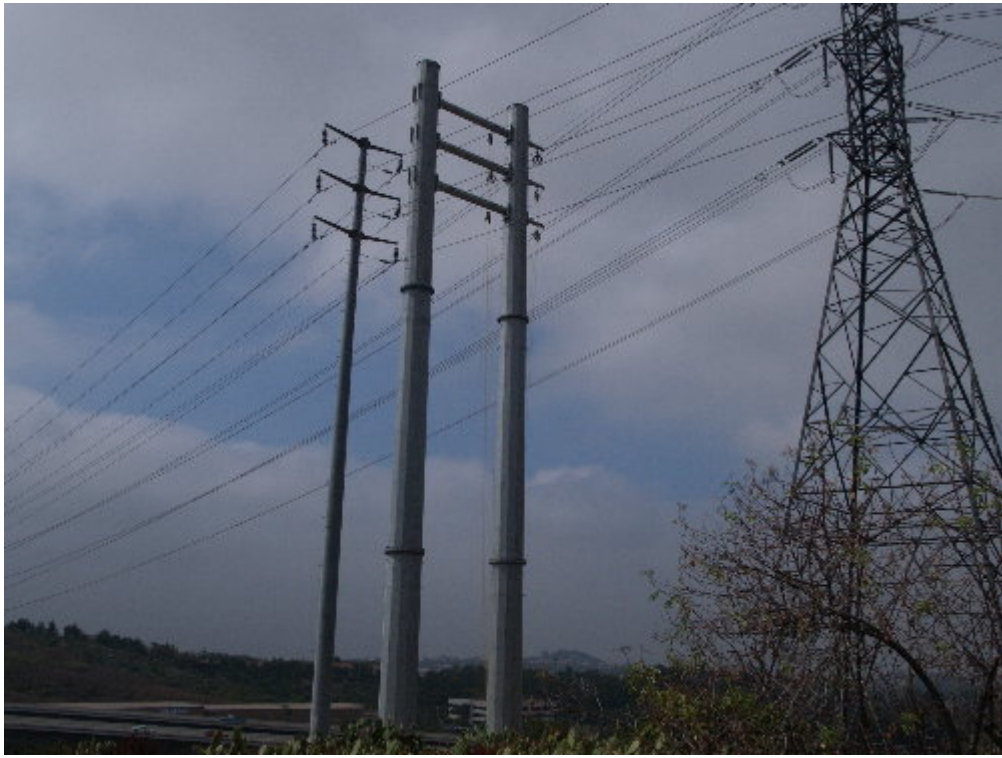
Figure 5 – H-structure 11 prepared for Saturday pull across the 241 toll road.
