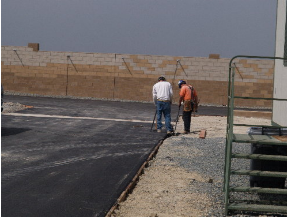
Figure 1 – The paving contractor repaired forms damaged by vehicle traffic.
