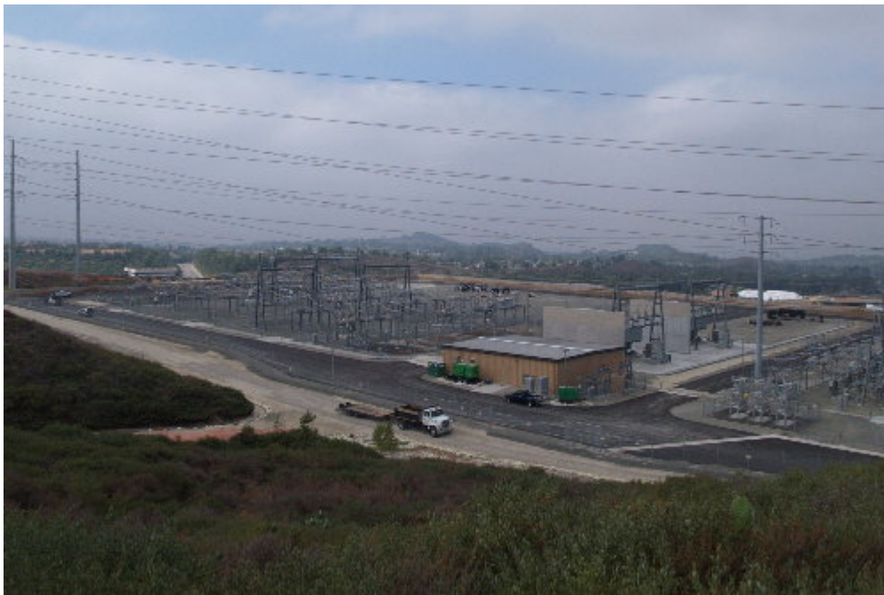
Figure 2 – Substation site after the paving on Saturday.
