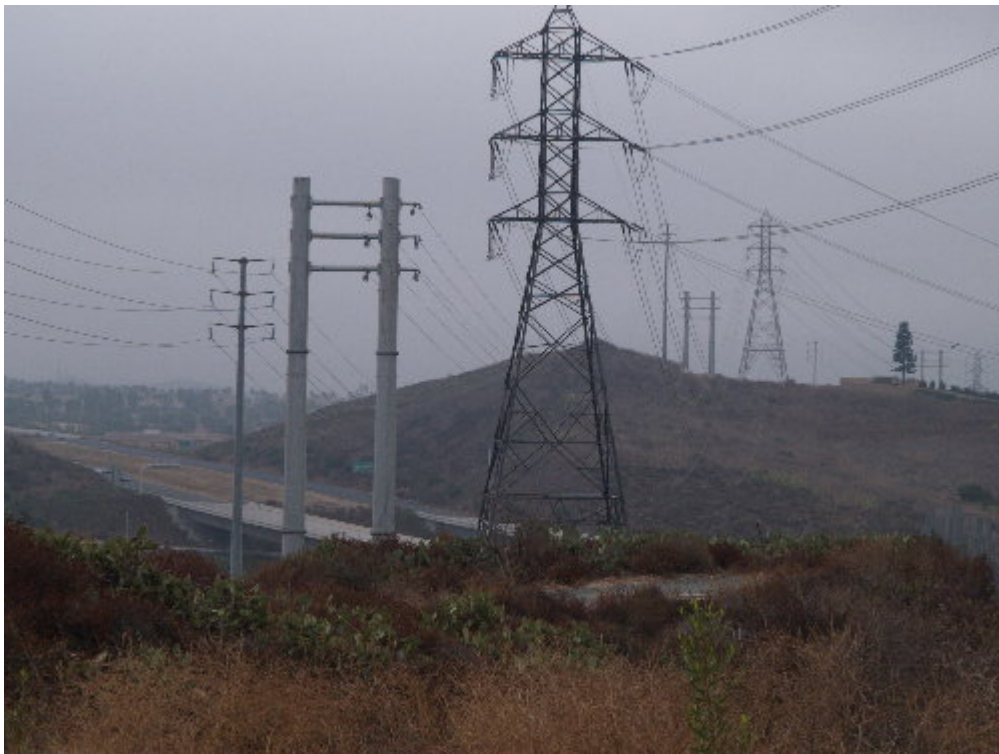
Figure 4 – H-Structure 11 to H-Structure 10 pull completed across the 241 toll road.
