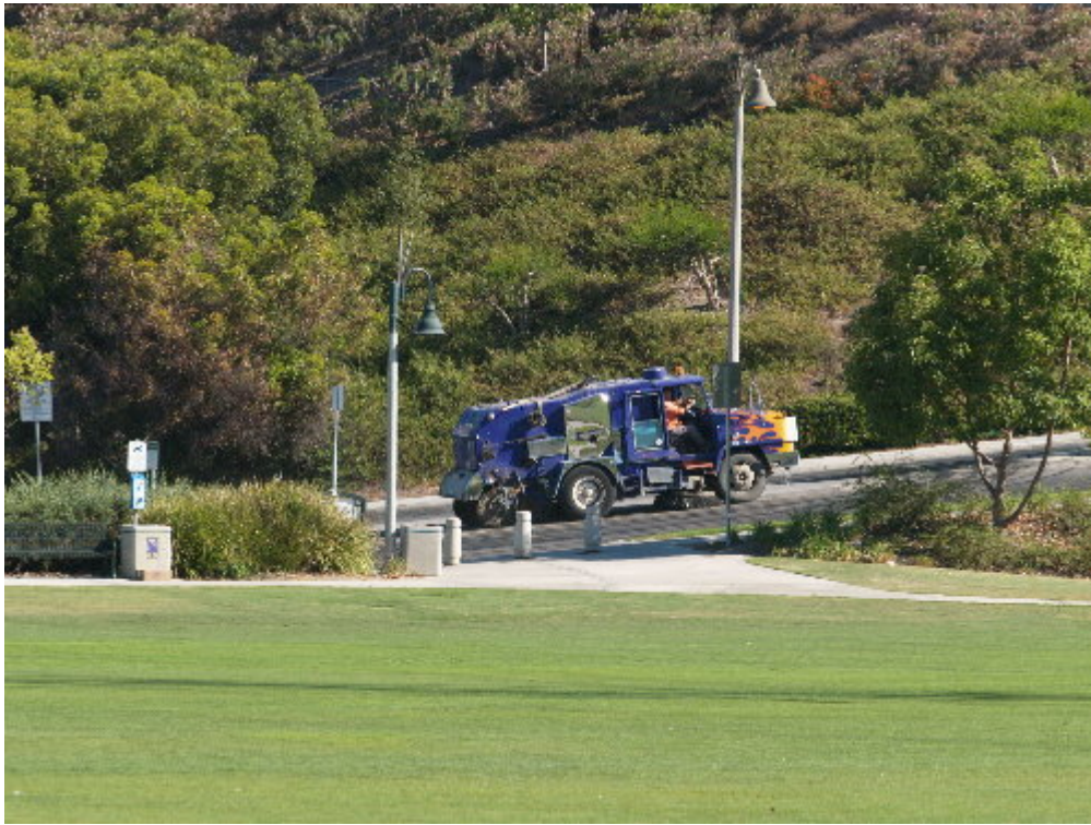
Figure 5 – A sweeper truck was used to clean the public right-of-way at the entrance to the access road.
