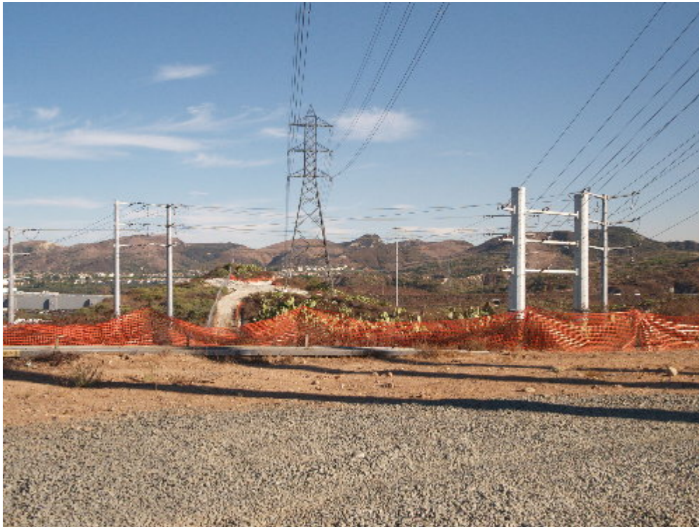
Figure 4 – Conductor has been pulled between the substation and H-structure 10.
