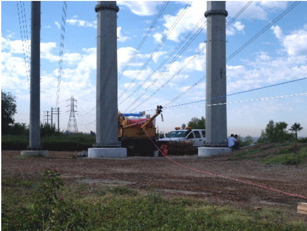
Figure 3 – The transmission crew set up to pull sock line.
