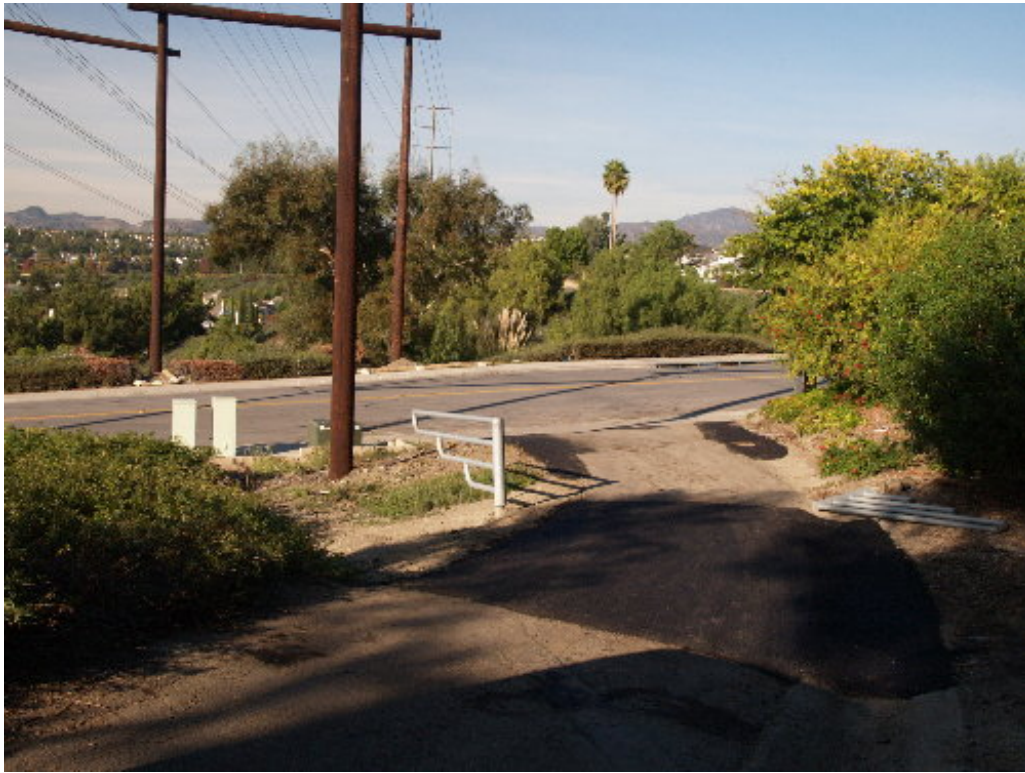
Figure 3 – The damage to the access road off La Barca done during construction has been repaired.
