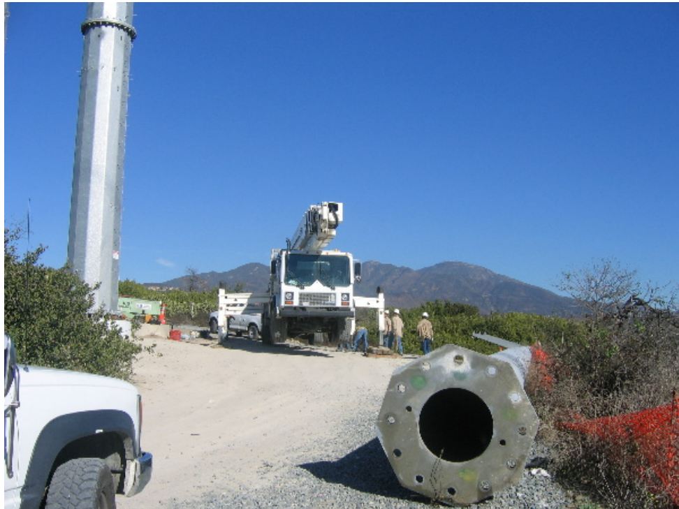
Figure 2 – Pole dismantling at Station M2-P2, near the Viejo Substation.
