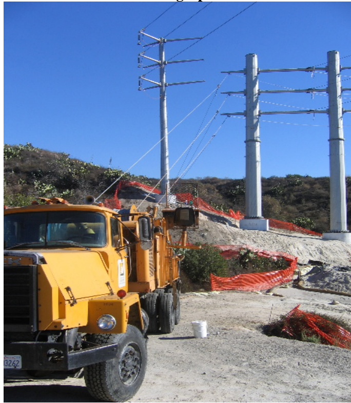
Figure 1 – Stringing activities at Tower HF-13
