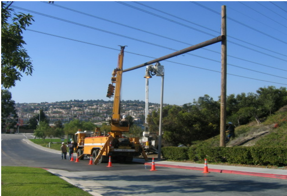
Figure 2 – Guard structure dismantling at Olympiad Road and Applegate, December 12, 2005.
