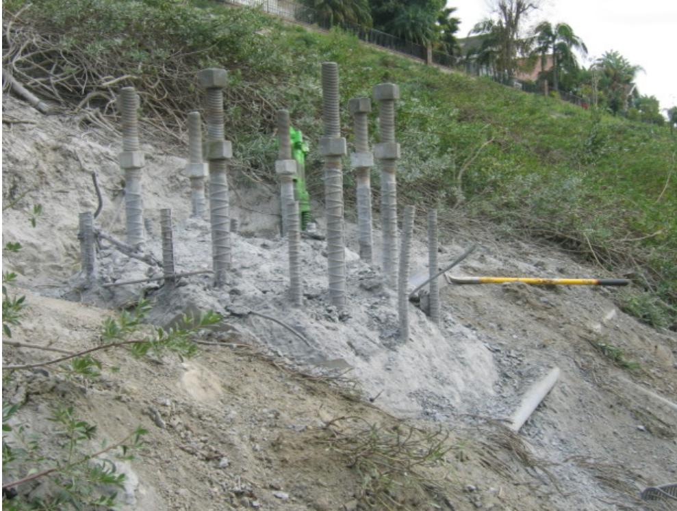
Figure 1 – Arizona Pipeline crew dismantling a tower footing by hand.
