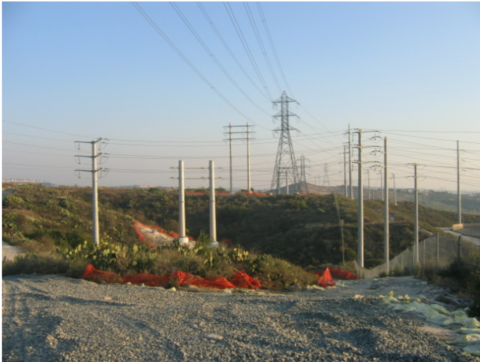
Figure 2 – Orange exclusion fencing around sensitive habitat near the new Substation.
