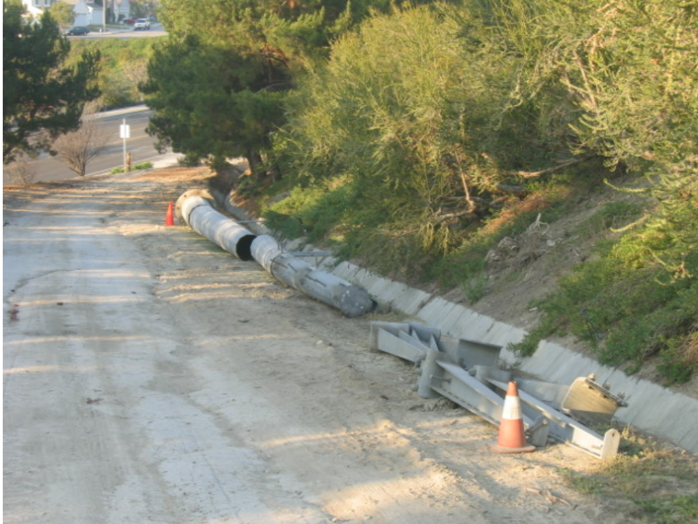
Figure 1 – Dismantled steel poles are cut up and removed from the right-of-way.
